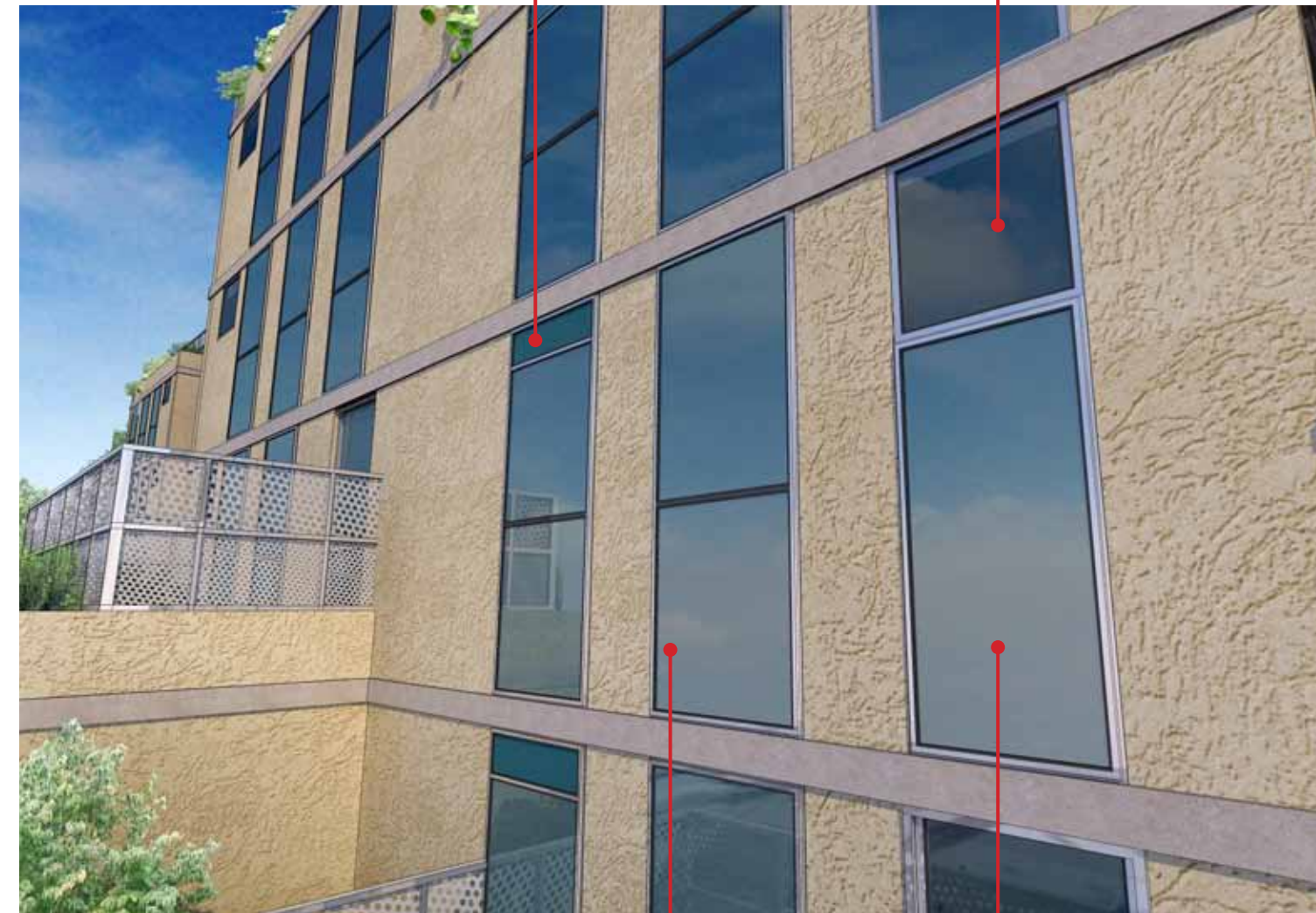
TYPICAL SPANDREL PANEL
