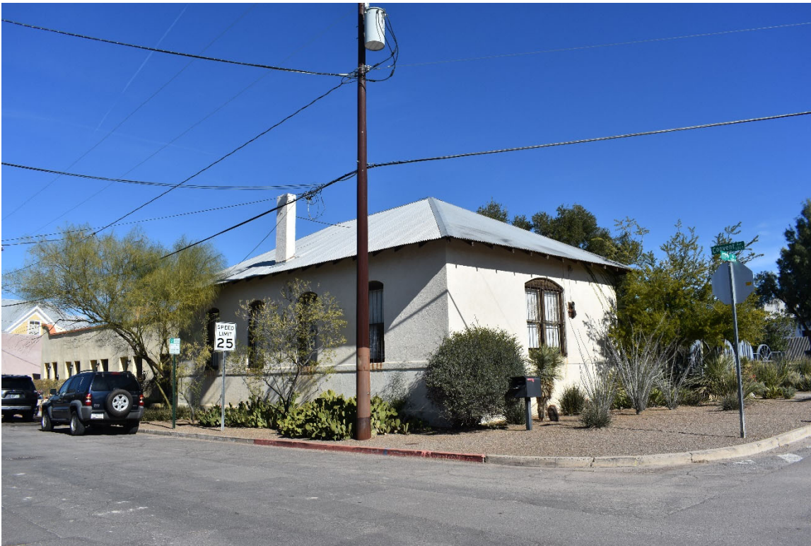
Figure 9. Old Prince Chapel African Methodist Episcopal (AME) Church. 531 South Convent Street showing west and south elevations. January, 2020.
