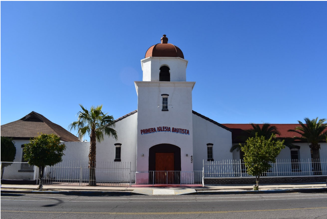
Figure53. Primeria Iglesia Bautista. 482 South Stone Avenue showing east elevation. January 2020.
