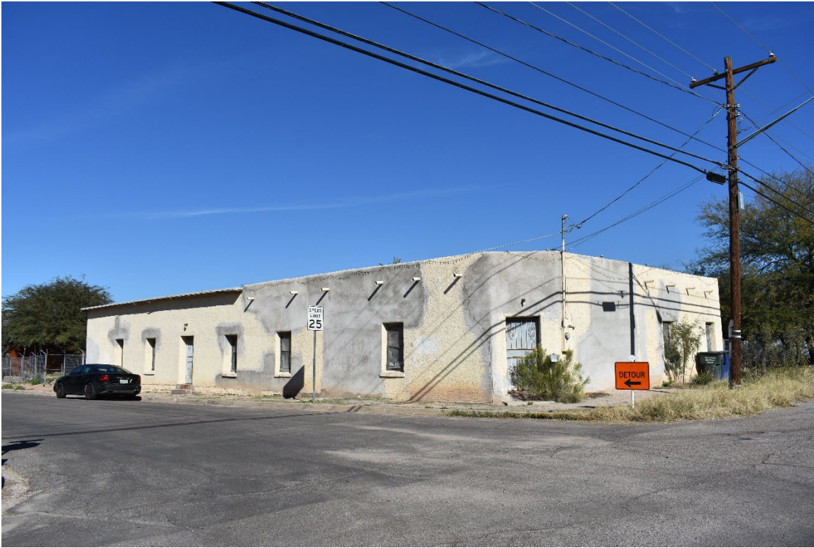
Figure 45. 685 South Meyer Avenue showing a modified example of a Classic Sonoran building with the characteristic chamfered entry of a commercial property. January 2020.
