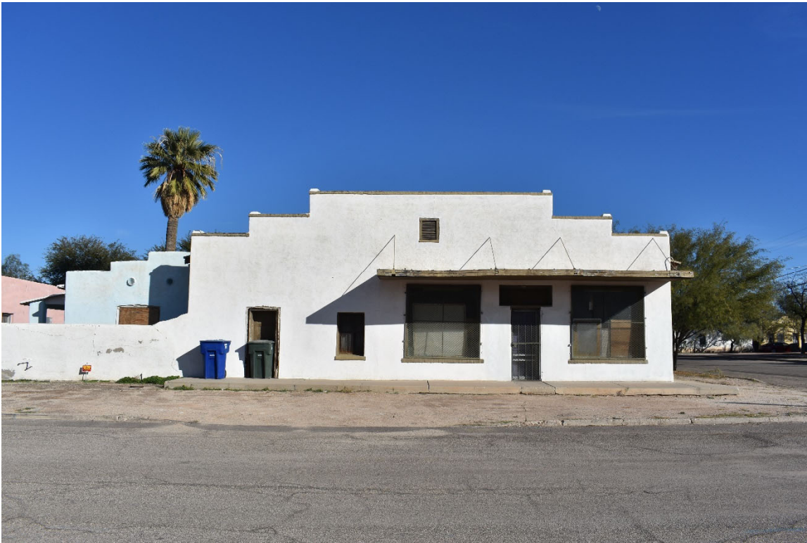
Figure 61. Former Gee Lung's Market. 863 South 9th Street showing an example of a one-part commercial block constructed from adobe masonry likely in the mid-1930s. January 2020.
