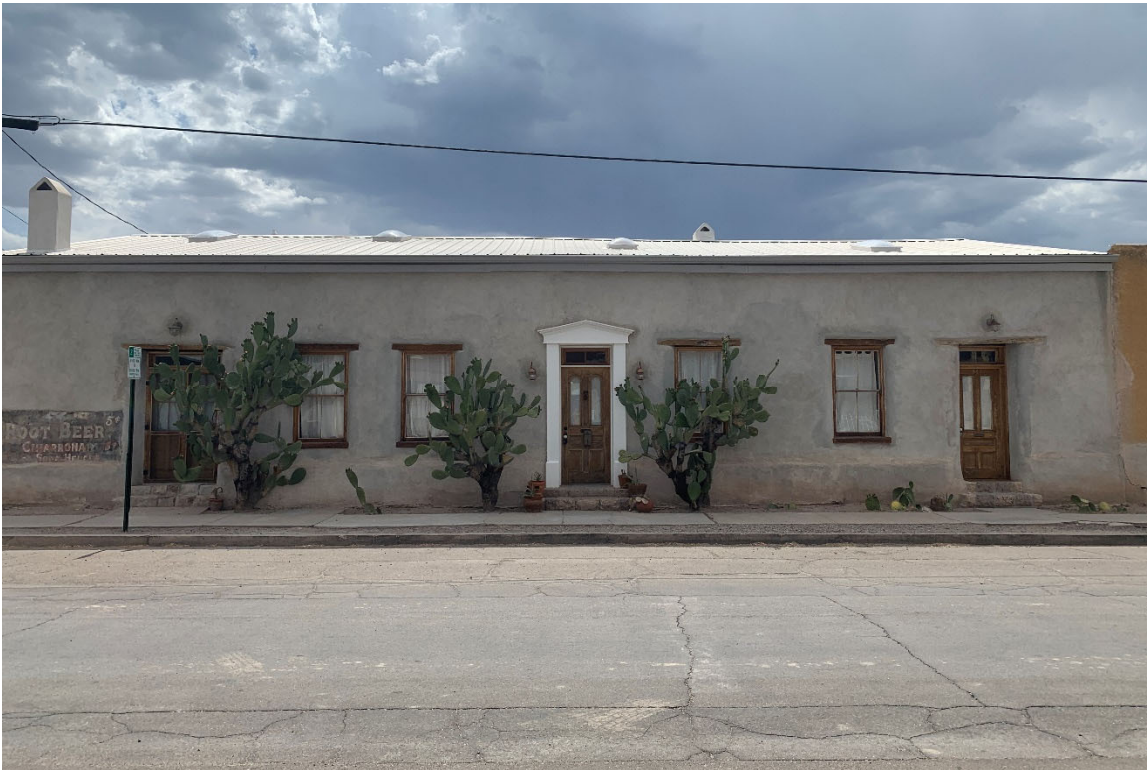
Figure 50. 506-512 South Meyer Avenue showing elements of the Italianate style on a Transformed Sonoran row house. The Italianate is most evident in the building's doors which show the use of paired glass panes and simplified classical surrounds. The style's influence is also evident in the two over two double hung sash windows. Note that this building has been heavily restored within the last decade and some of these elements may not be original. May 2020.
