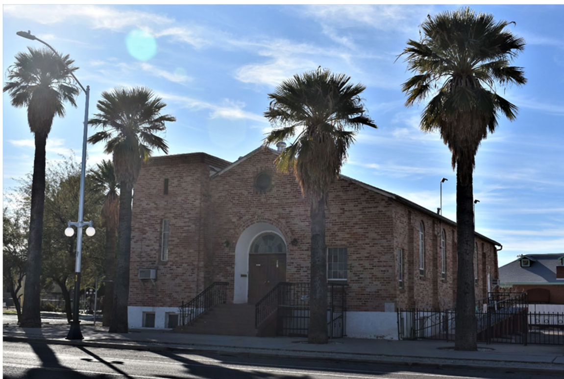
Figure 14. Prince Chapel African Methodist Episcopal (AME) Church. 602 South Stone Avenue showing east and north elevations. January 2020.
