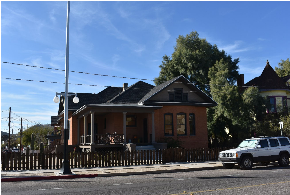
Figure 49. 396 South Stone Avenue showing a Queen Anne style residence. January 2020.
