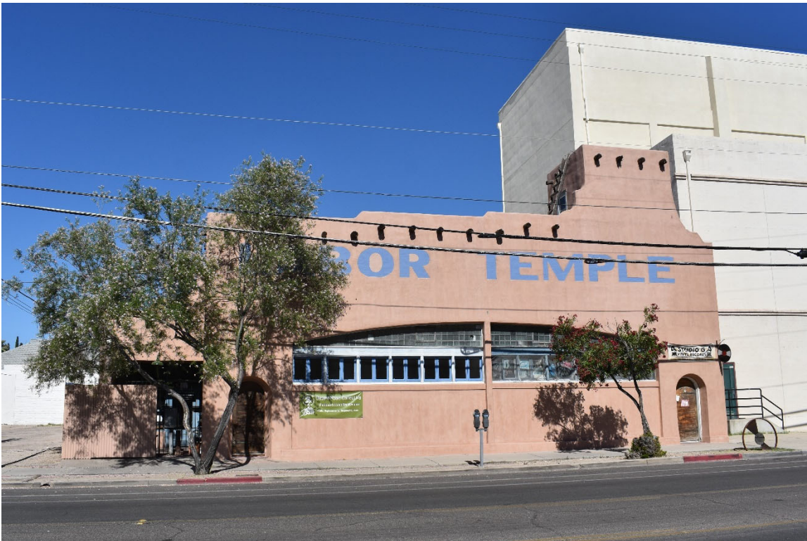
Figure 66. Labor Temple. 267 South Stone Avenue showing west elevation. Note the decorative ladder connecting the roof of the second and third story. See also Figure 56. May 2020.
