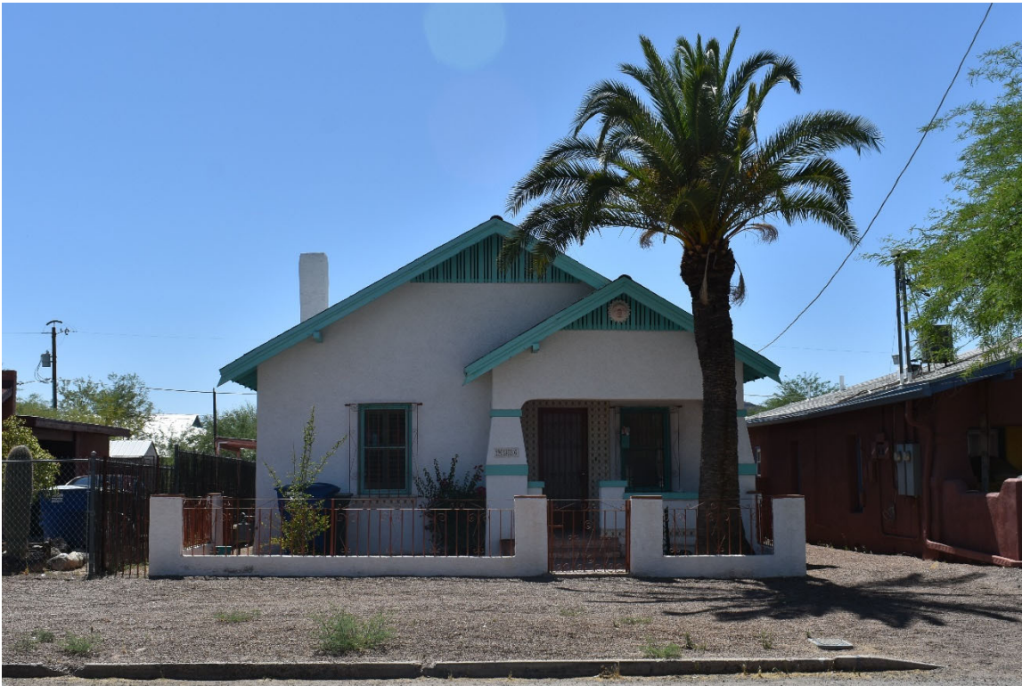
Figure 57. 930 South 8th Avenue showing an example of a front-gabled craftsman bungalow constructed from adobe masonry. May 2020.
