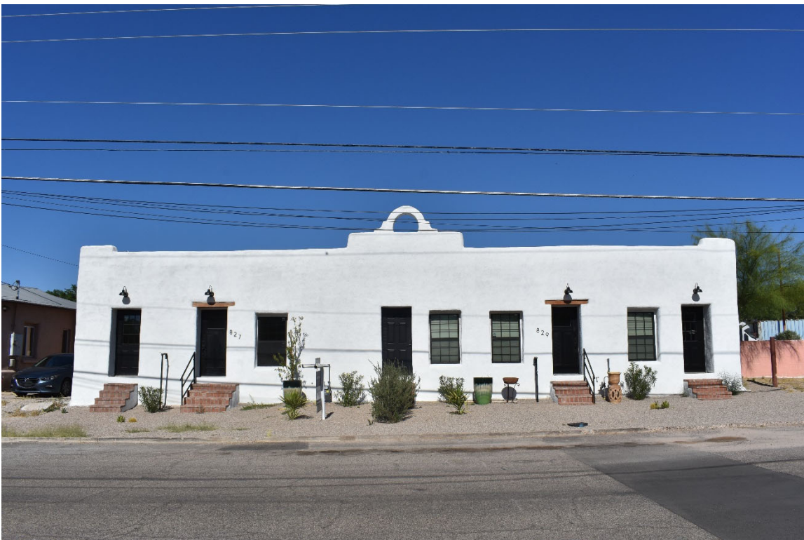
Figure 52. 827-829 South 8 th Avenue showing several row houses incorporating elements of the Mission Revival style including a decorative parapet and white walls. May 2020.
