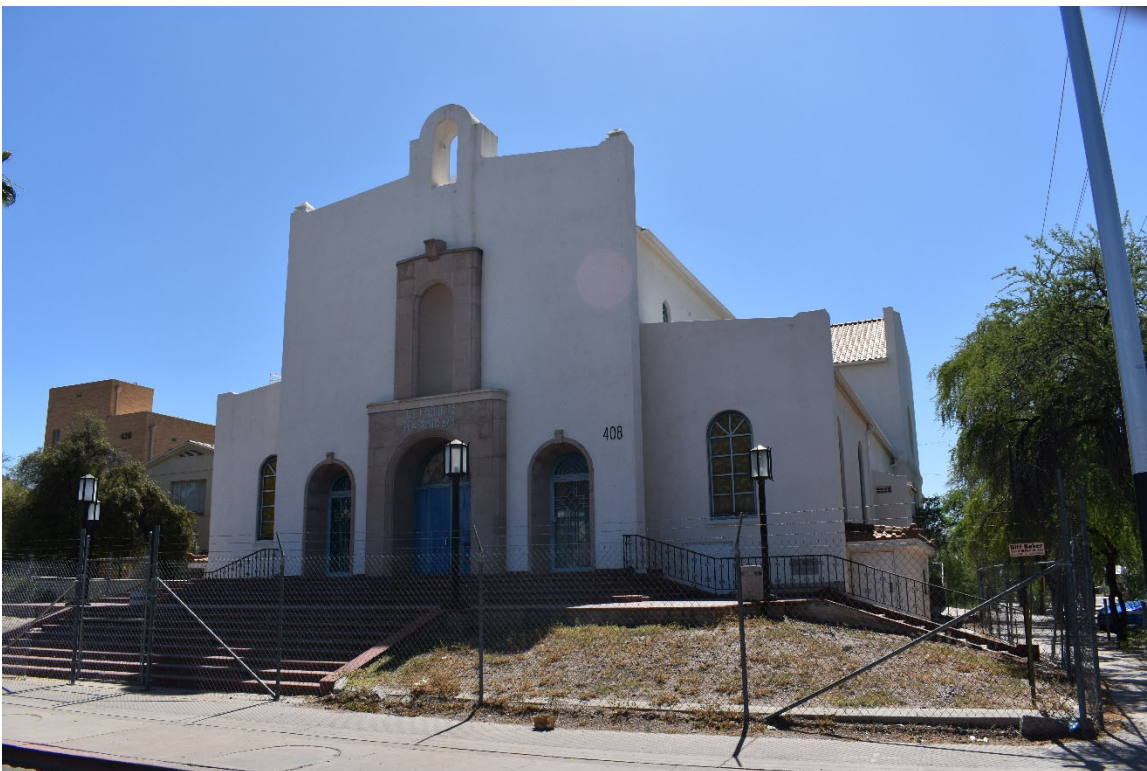
Figure 62. All Saints Church. 408 South 6 th Avenue showing north and east elevations. May 2020.
