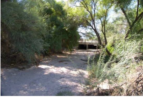
Photo 3: Looking at Rose Hill Wash crossing under Speedway Boulevard.
