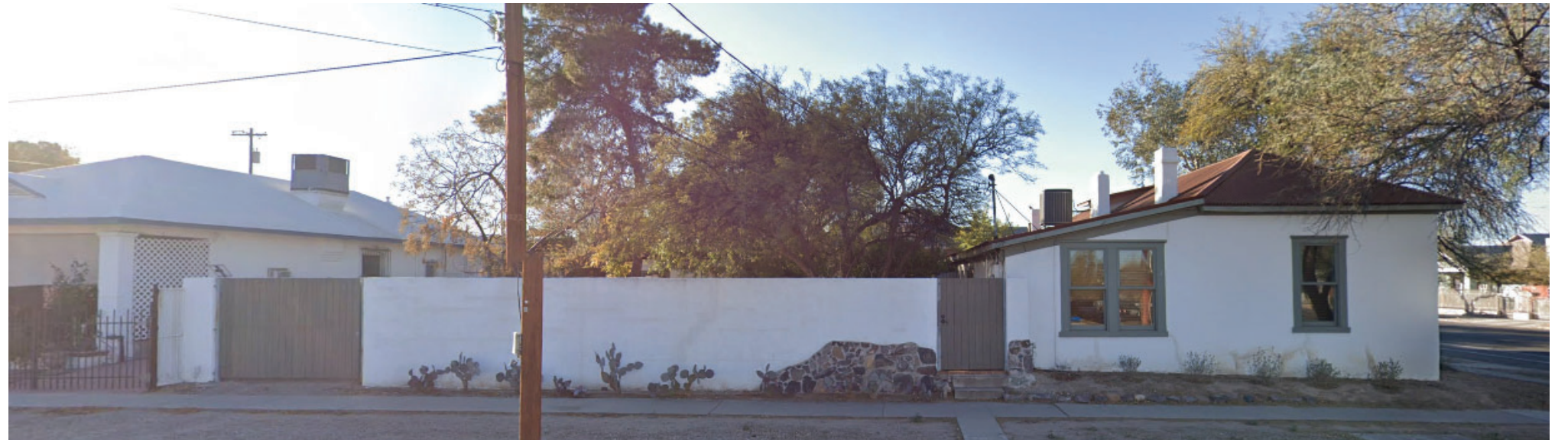
View from North Looking South
