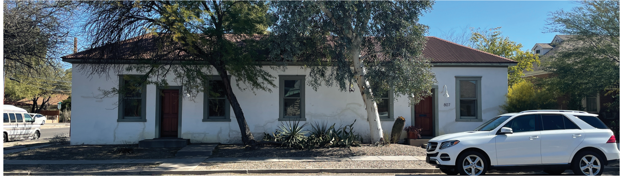
View of West Facade Windows and Doors
