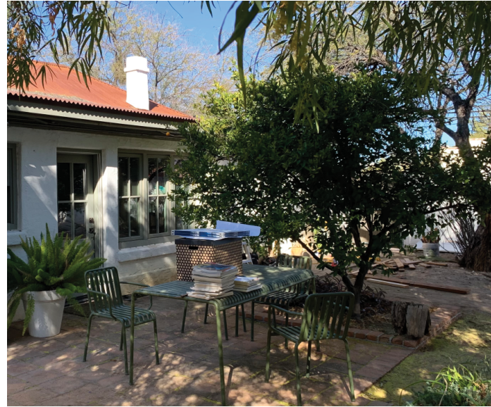
View of East Facade Windows and Door
