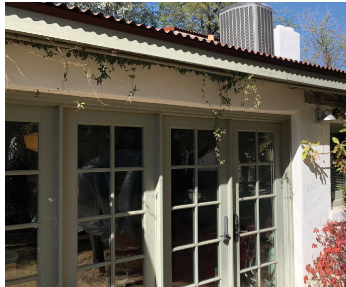
View of East Facade Windows and French Door
