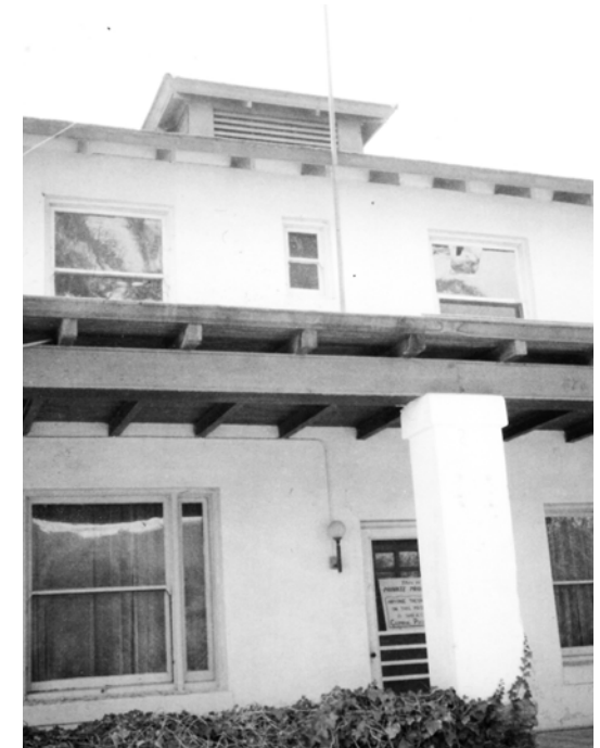
North Elevation detail
