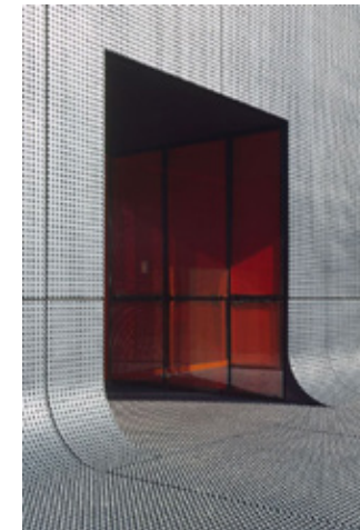
Curved ground plane. Plaza curving up to become part of the building.
