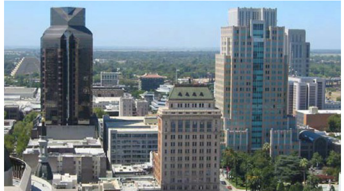
Figure 4-83. View of the Central Core, from the top of the Empire Building, looking west. These buildings employ a variety of stepback strategies, ranging from stepbacks only at the top to frequent stepbacks applied at various stages of as the buildings rise.
