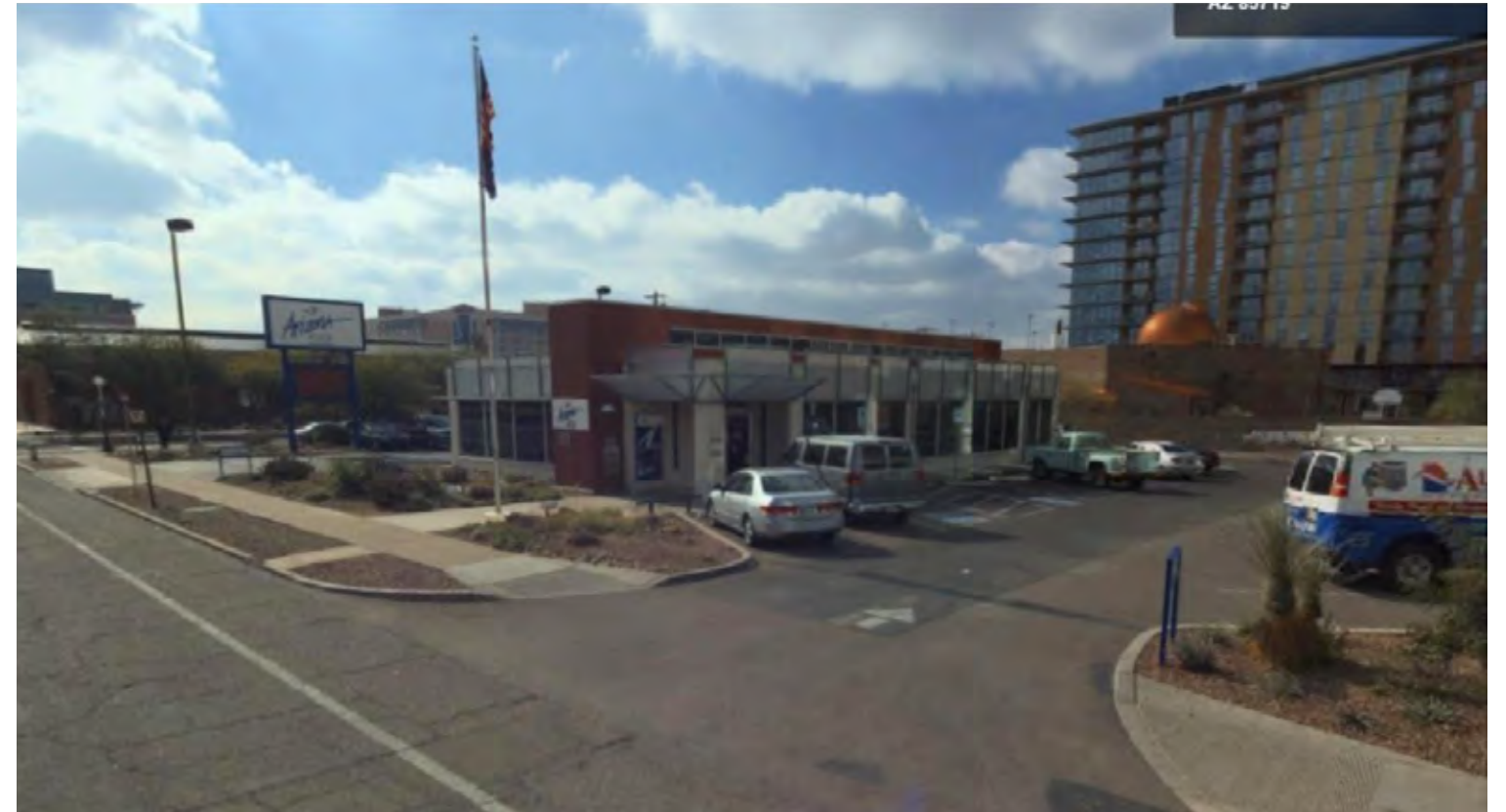
PARK AVENUE LOOKING SOUTH-WEST
