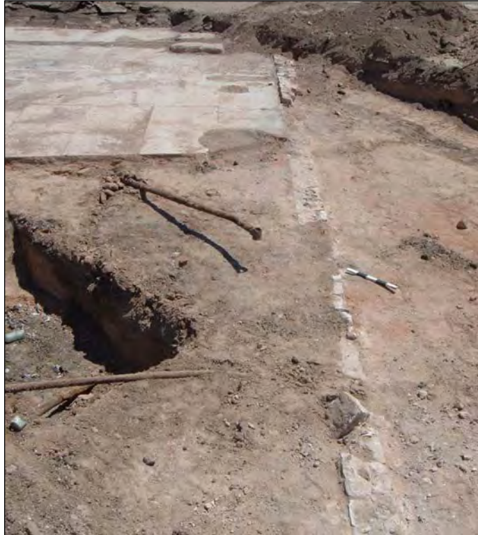
Figure 27. Northern portion of Feature 76, including concrete slab. The northwestern foundation wall of Feature 52 is visible on the right.
