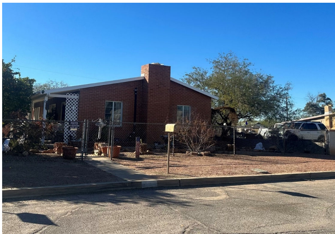
Photo 6. 630 South Santa Rita Avenue, view facing northwest (WestLand, January 2023 [AZ_PimaCounty_BarrioSanAntonio_0006])
