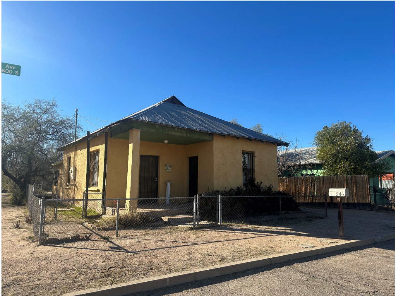
Photograph 3. 546 South Star Avenue, view facing northwest. (WestLand Engineering & Environmental Services, January 2023 [AZ_PimaCounty_BarrioSanAntonio_0003] jpeg).
