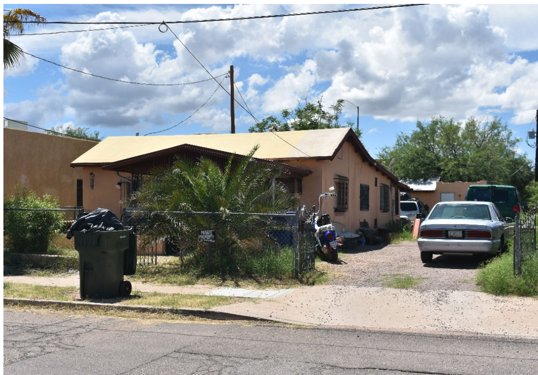
Photo 7. Example of building additions to the rear of 506 S. Fremont Avenue, view facing southwest (WestLand, January 2023 [AZ_PimaCounty_BarrioSanAntonio_0006])
