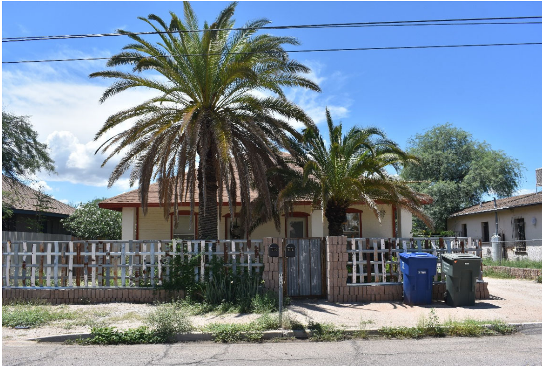
Photo 8. Example of fencing at 416 S. Fremont Avenue, view facing west (WestLand, January 2023 [AZ_PimaCounty_BarrioSanAntonio_0008])
