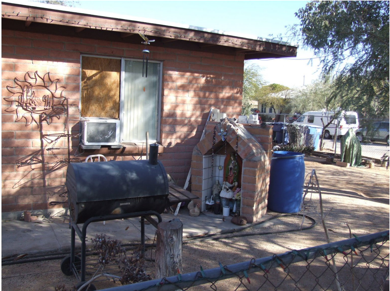
Photograph 9. Example of a yard shrine at 546 S. Santa Rita Avenue, view facing northeast. (WestLand Engineering & Environmental Services, January 2023 [AZ_PimaCounty_BarrioSanAntonio_0009] jpeg).
