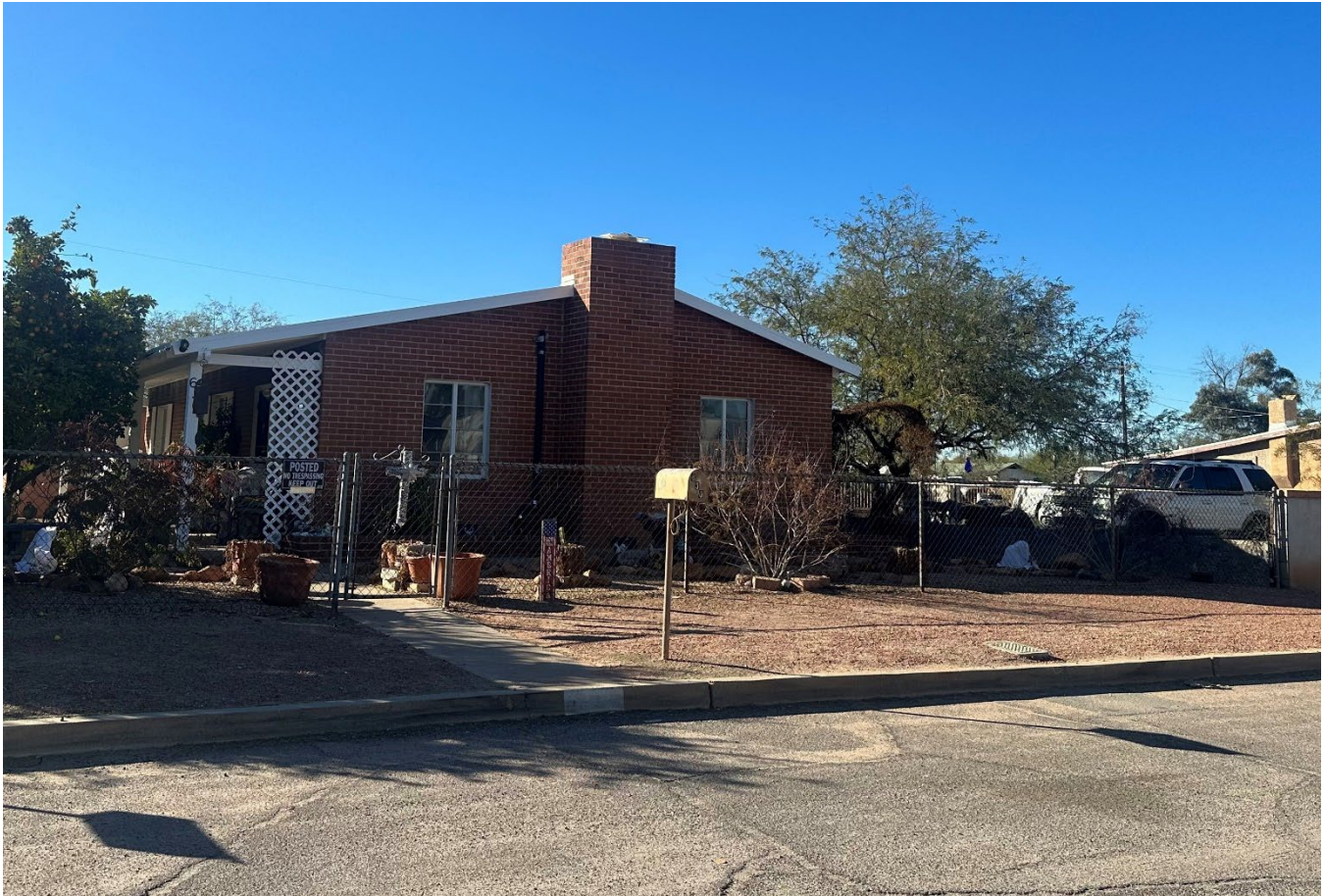
Photograph 6. 630 South Santa Rita Avenue, view facing northwest. (WestLand Engineering & Environmental Services, January 2023 [AZ_PimaCounty_BarrioSanAntonio_0006] jpeg).
