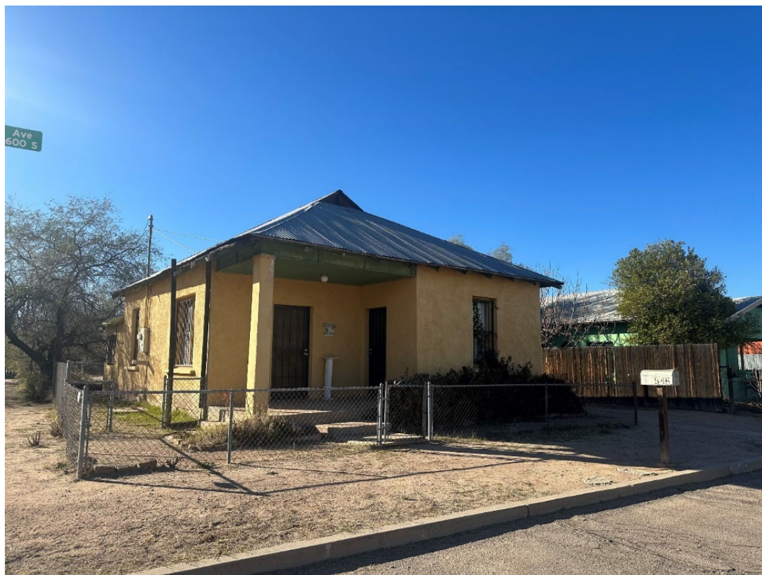
Photo 3. 546 South Star Avenue, view facing northwest (WestLand, January 2023 [AZ_PimaCounty_BarrioSanAntonio_0003])
