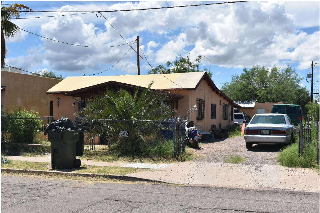
Photograph 7. Example of building additions to the rear of 506 S. Fremont Avenue, view facing southwest. (WestLand Engineering & Environmental Services, January 2023 [AZ_PimaCounty_BarrioSanAntonio_0007].jpeg).
