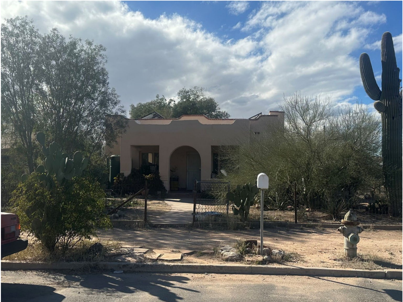
Photograph 5. 402 South Star Avenue, view facing west. (WestLand Engineering & Environmental Services, January 2023 [AZ_PimaCounty_BarrioSanAntonio_0005].jpeg).
