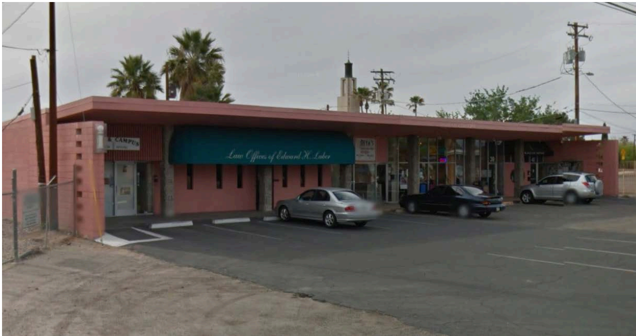
Fig. 19. Boulevard Shops, Sunshine Mile, 33- 41 North Tucson Blvd. Nicholas Sakellar, architect. Photo: Google, 2013.
