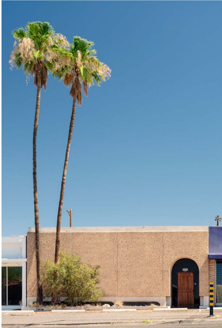
Fig. 27. Friedman Office Building, (1950, 1965 & 1967), Photo by GMVargas 2017.
