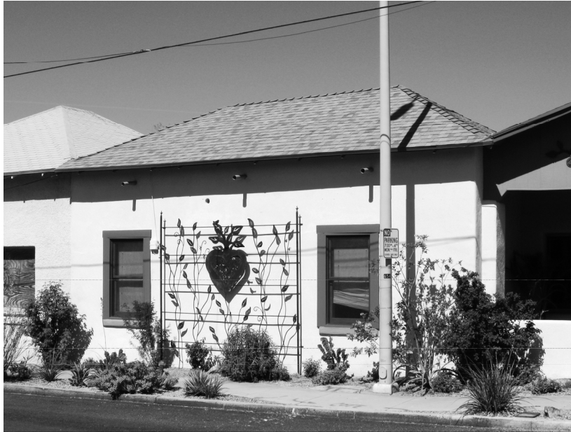
Photograph 21. 656 N. Anita Ave., view northeast.
