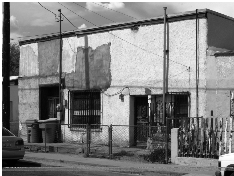
Photograph 16. 926 N. Anita Ave.; view east-northeast.
