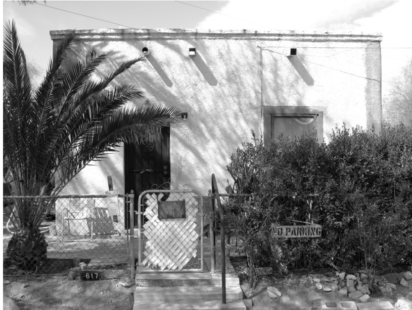
Photograph 1. 617 N. Brady Ave.; view west-southwest.
