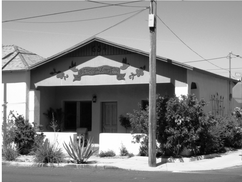
Photograph 5. 654 N. Anita Ave.; view northeast.
