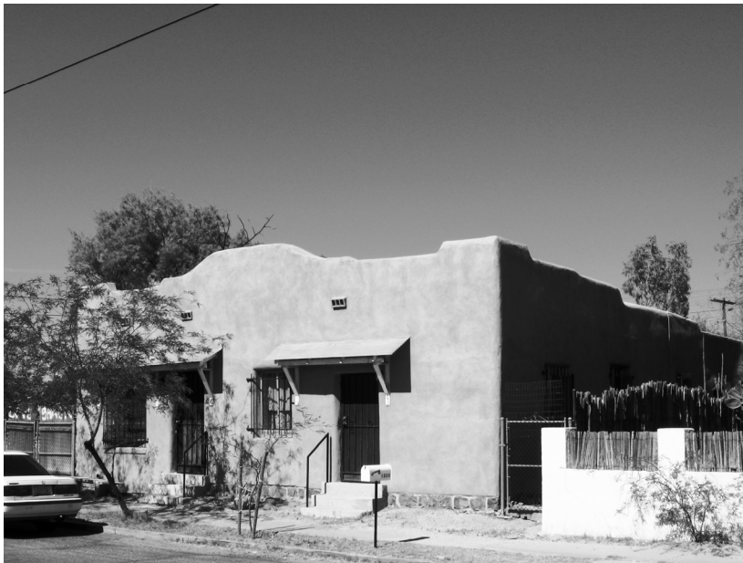
Photograph 22. 1000 N. Anita Ave.; view north-northeast.
