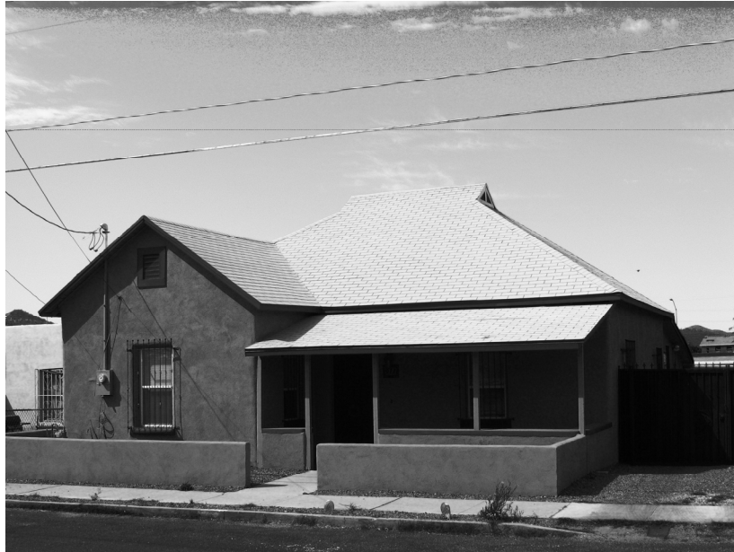
Photograph 3. 911 N. Anita Ave.; view southwest.
