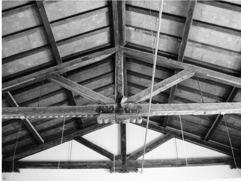
Photograph 25. Oury Center, 600 W. St. Mary's Rd.; interior, view north-northeast.
