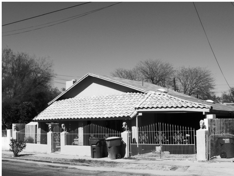
Photograph 14. 940 N. Anita Ave.; view northeast.
