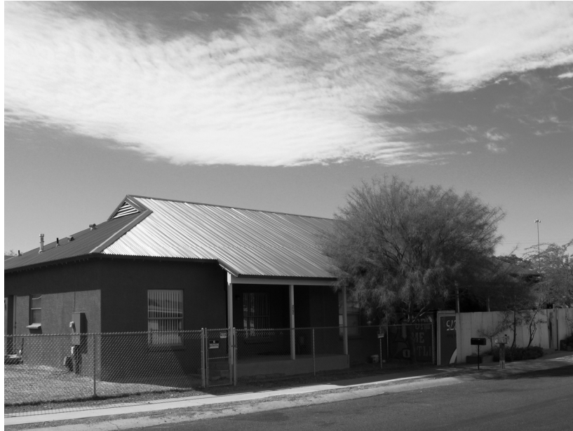
Photograph 13. 545-547 W. Shibell St.; view south.
