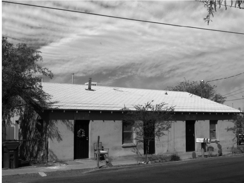
Photograph 23. 709-713 N. Anita Ave.; view west-northwest.
