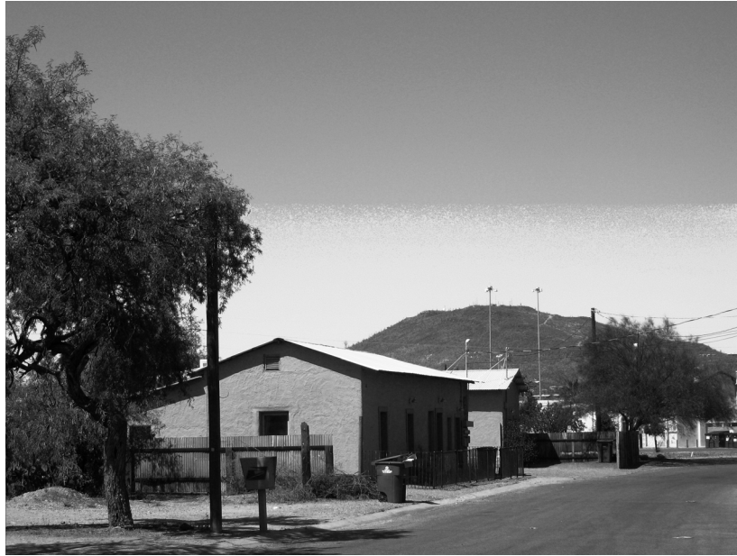
Photograph 11. W. Oury St. between W. Hughes St. and N. Anita Ave.; view southwest.
