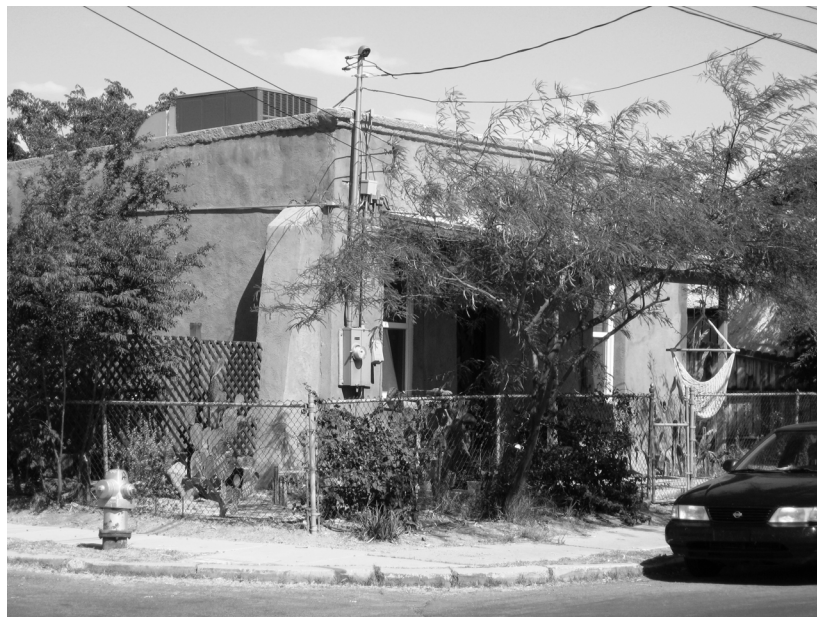
Photograph 24. 798 N. Contzen Ave.; view east-southeast.
