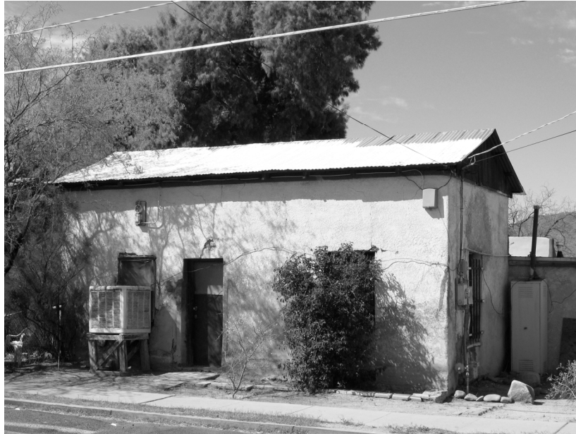
Photograph 19. 673 N. Anita Ave.; view southwest.
