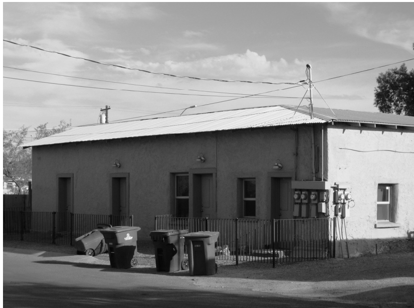
Photograph 2. 515 W. Oury St.; view southeast.
