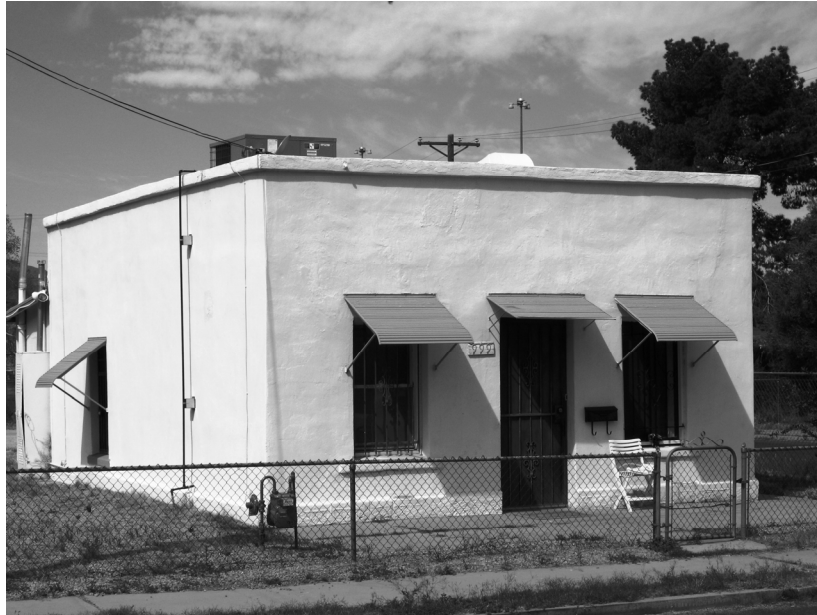
Photograph 17. 999 N. Anita Ave.; view west-northwest.
