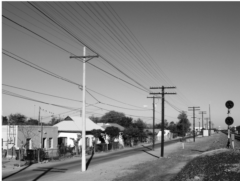
Photograph 12. N. Van Alstine Ave. between W. Oury St. and W. Speedway Blvd.; view northwest.
