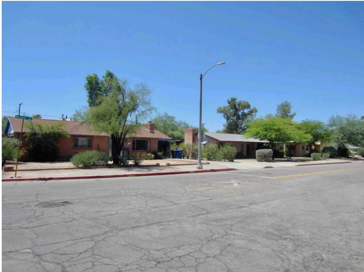
Photo 1 View of Manchester Street from the intersection with Eastbourne Ave., looking southwest. 2019
