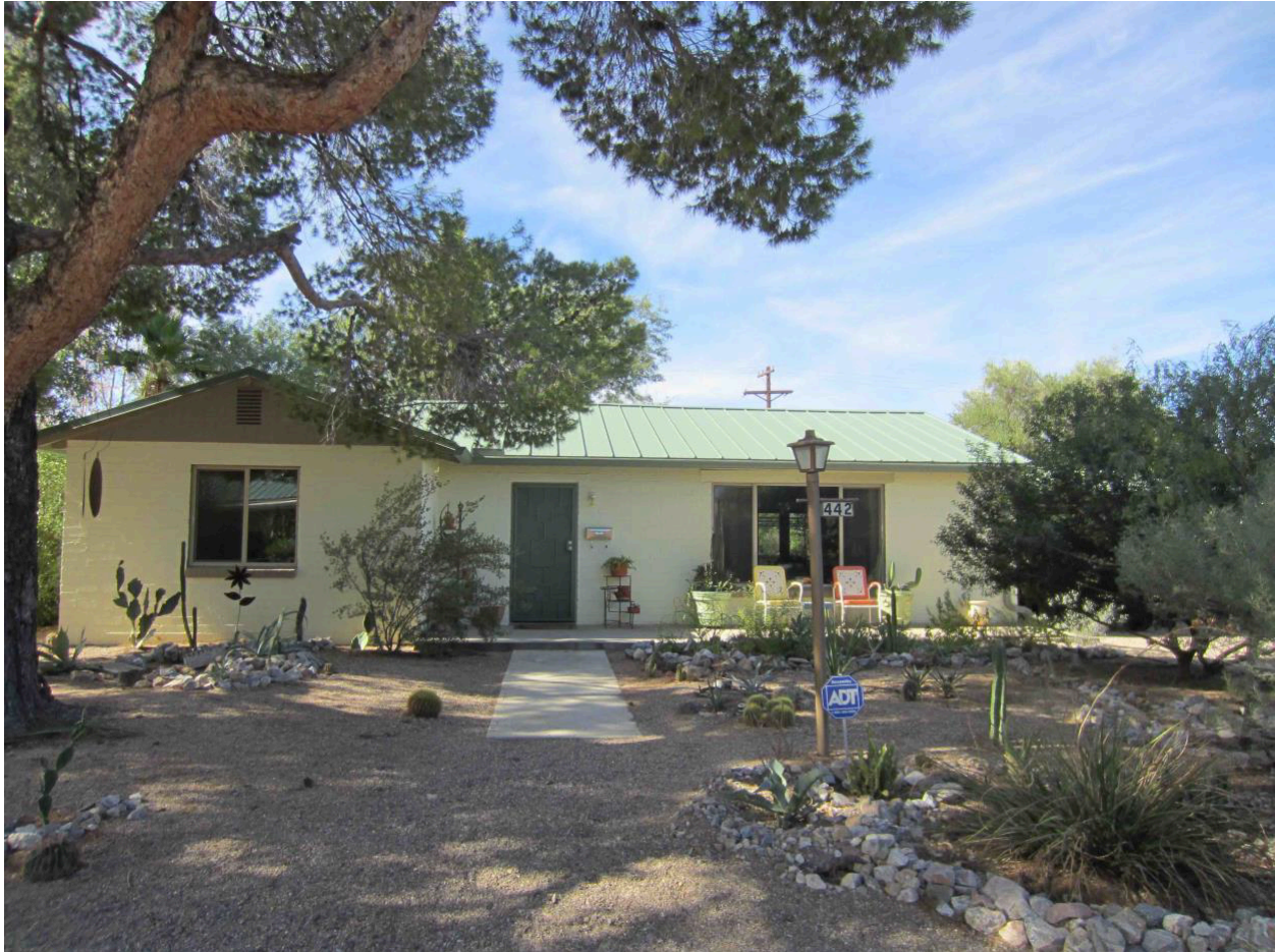
Photo 25 Example of a non-contributor at 442 S. Stratford Ave. The windows have been replaced and roofing materials modified. 2018.
