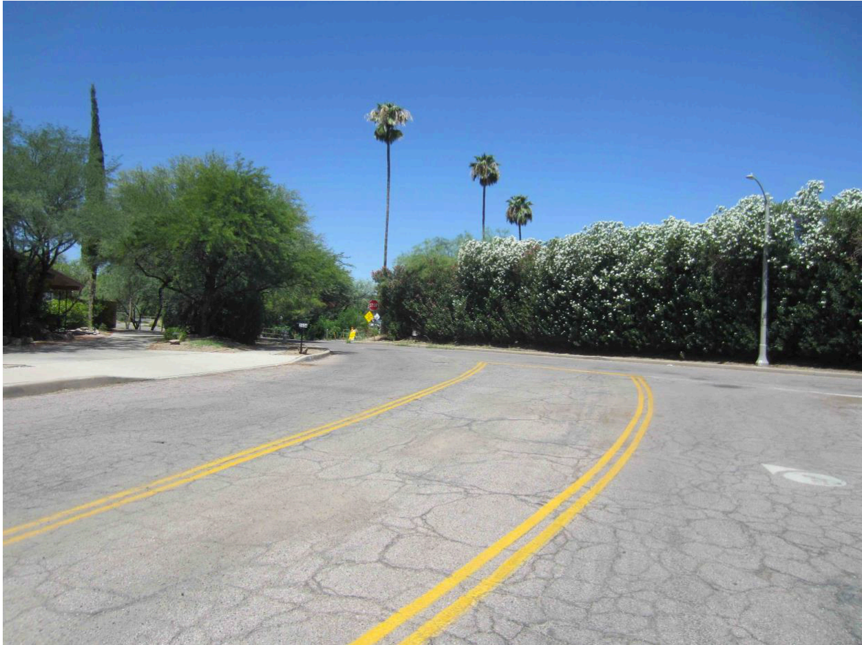
Photo 6 View of oleanders along Arroyo Chico drainageway from the intersection of Stratford Ave., looking north. 2019.
