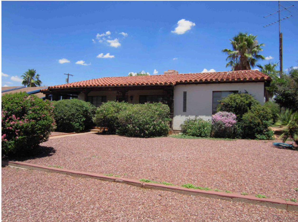
Photo 21 Spanish Colonial Ranch house located at 2615 E. Devon Street. 2019.
