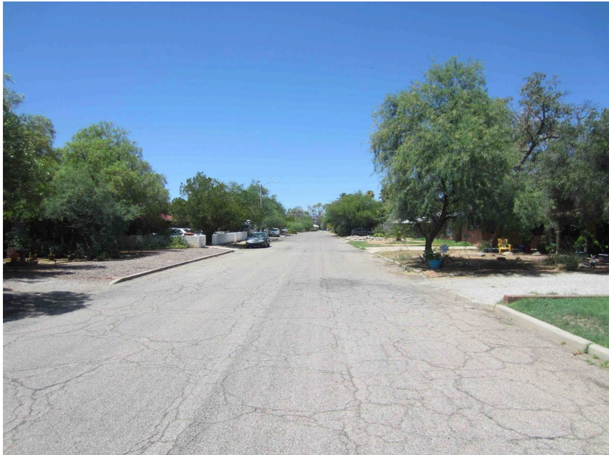
Photo 5 View of Croyden Street, looking west. 2019.
