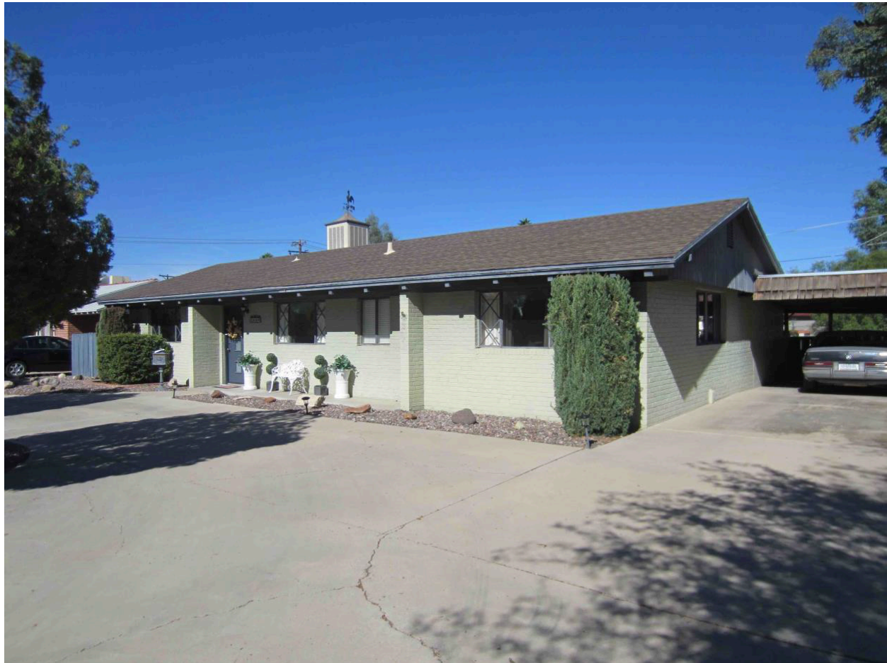
Photo 20 Ranch house located at 2809 E. Malvern Street. 2018.
