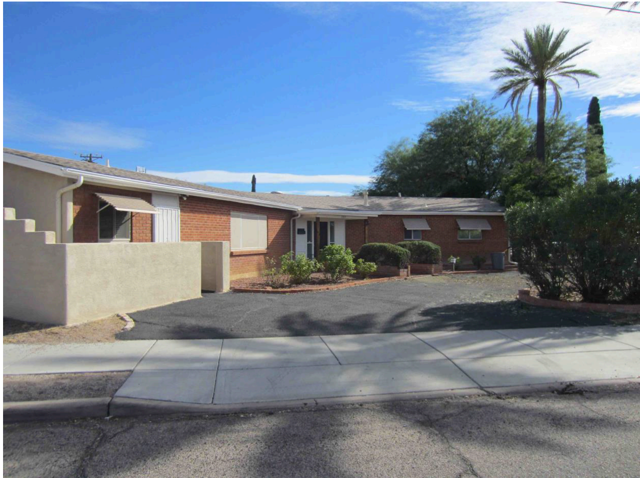
Photo 24 Example of a non-contributor at 2801 E. Manchester Street. The windows have been replaced, carport converted to interior space, and a patio wall has been added. 2018.
