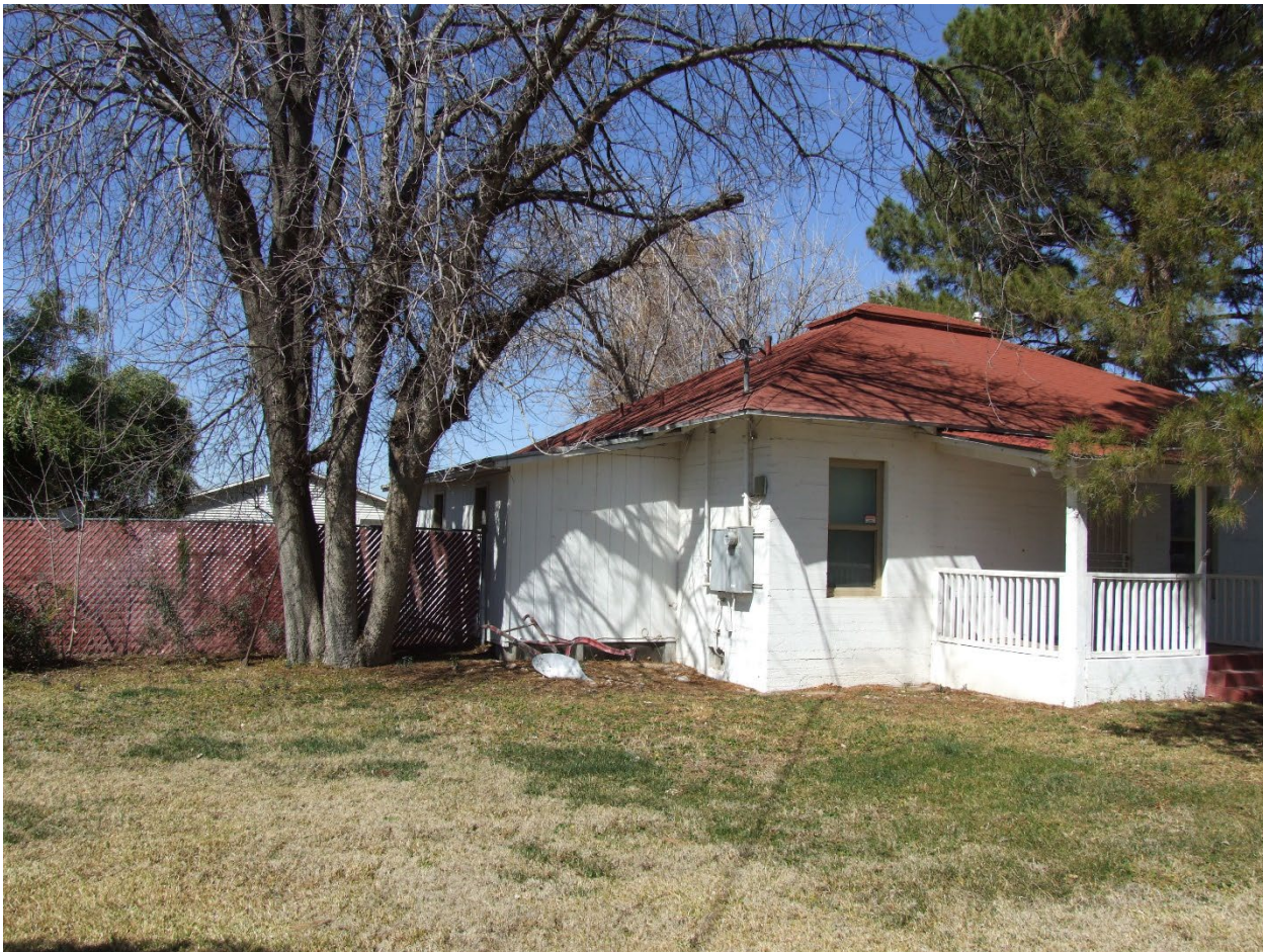
The University of Arizona Campus Agricultural Center, Main Residence, east and south elevations, view facing northwest. WestLand Resources, Inc., March 8, 2023.
