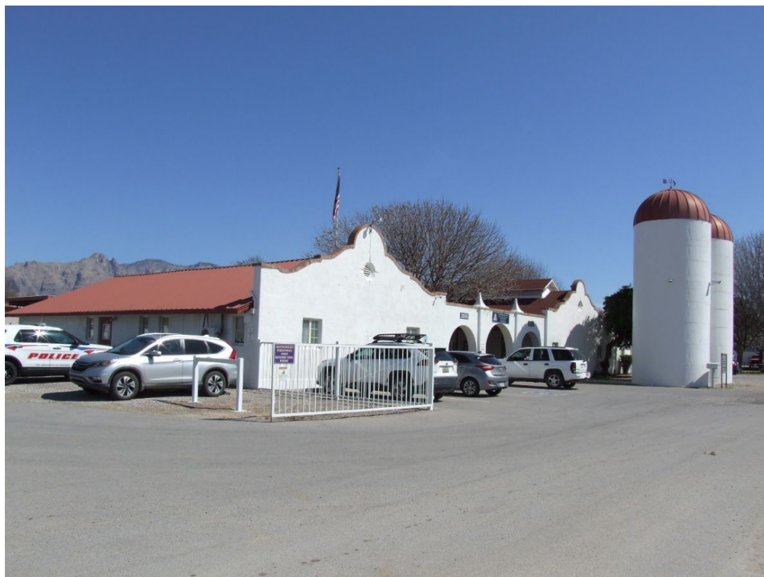
Photograph 18. West and south elevations of the Classroom Building; view facing northeast (AZ_Pima County_UA Campus Agricultural Center Historic District_0018)
