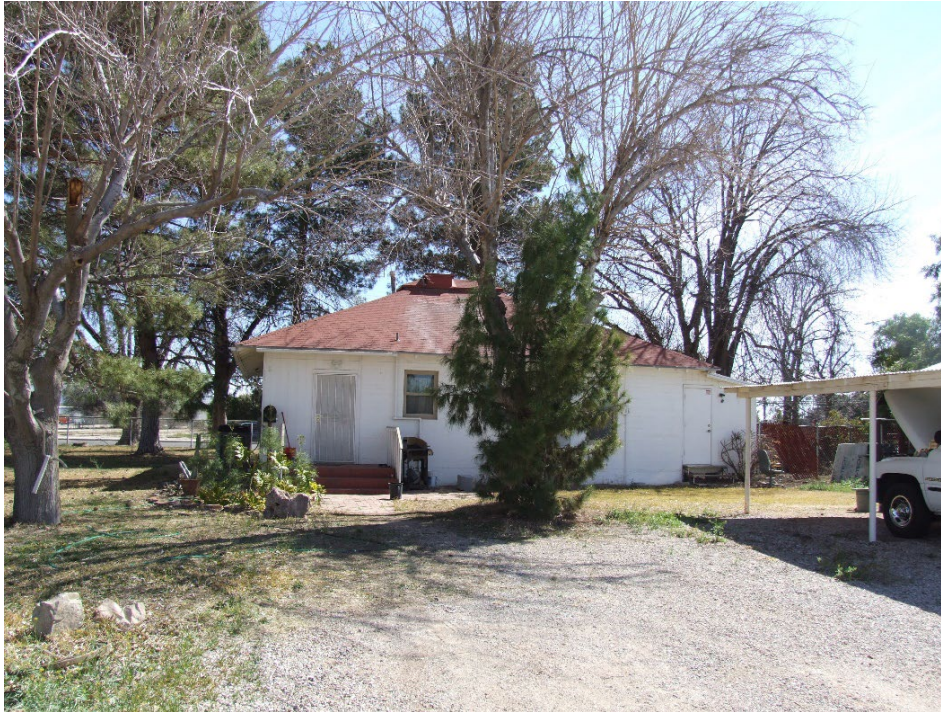
Photograph 5. West elevation of the Residence and back entryway; view facing east (UA_Pima County_UA Campus Agricultural Center Historic District_0005)
