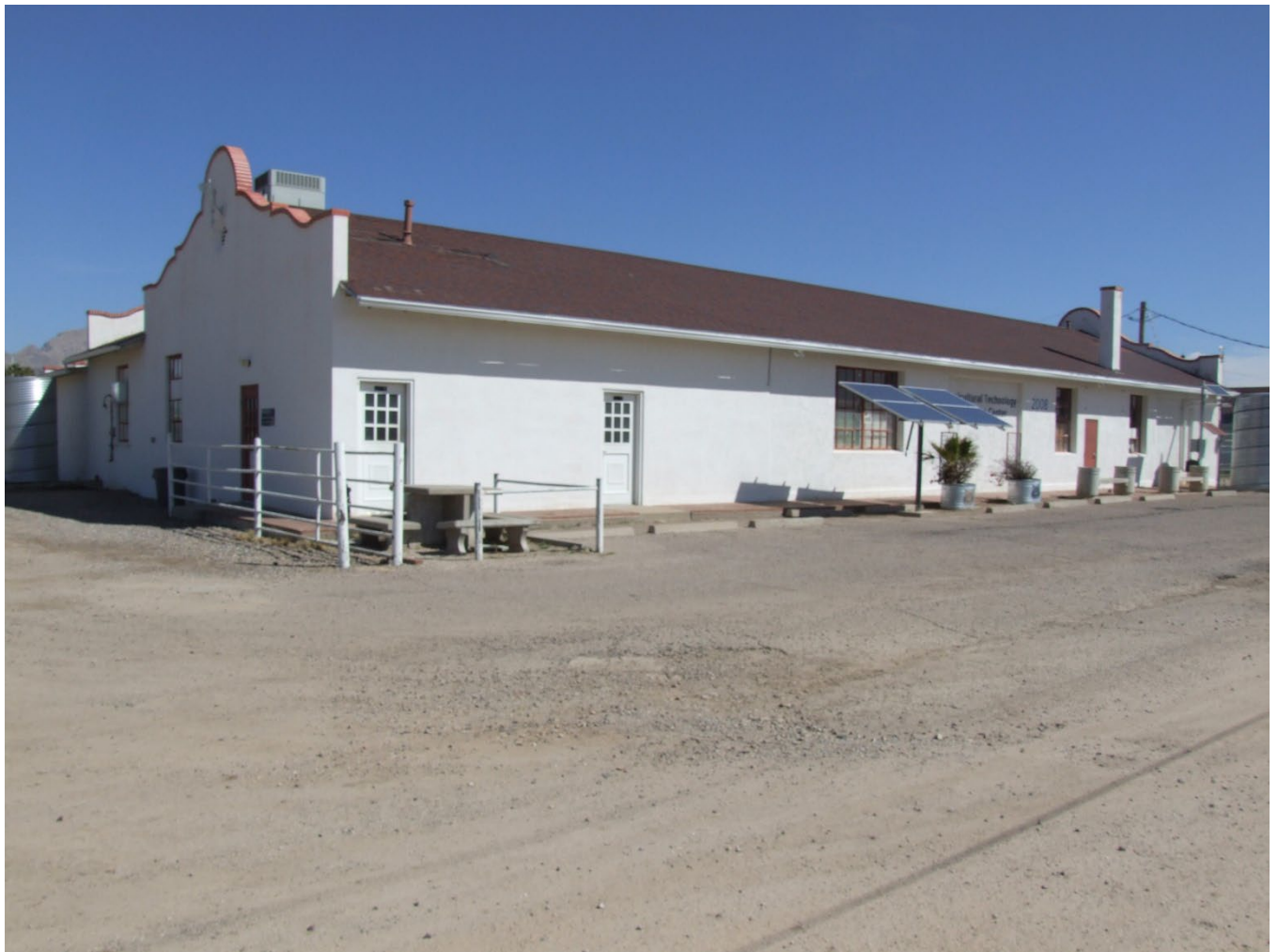
The University of Arizona Campus Agricultural Center, Agricultural Education Facility Building, view facing northeast. WestLand Resources, Inc. March 8, 2023.
