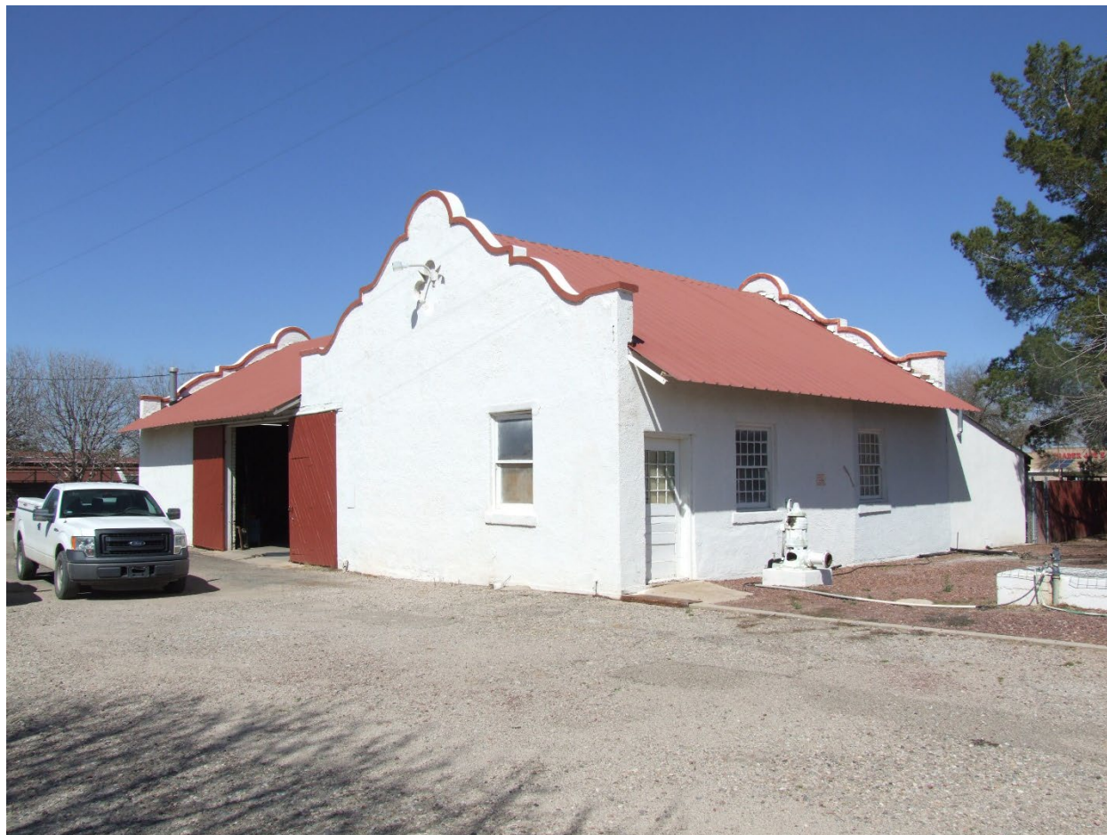
Photograph 10. East and south elevations of the Machine Shop; view facing northwest (AZ_Pima County_UA Campus Agricultural Center Historic District_0010)
