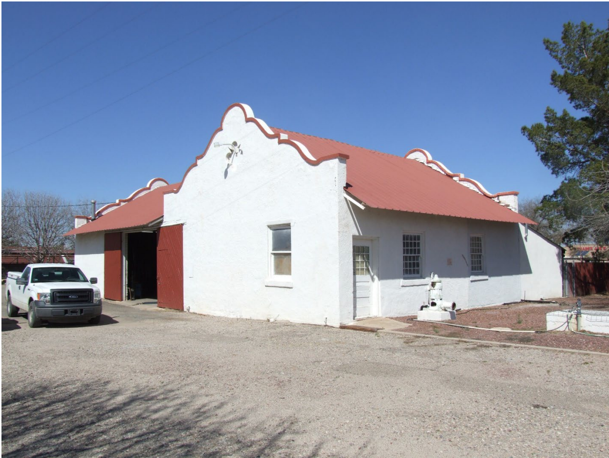
The University of Arizona Agricultural Center, Machine Shop, view facing northwest. WestLand Resources, Inc., March 8, 2023.
