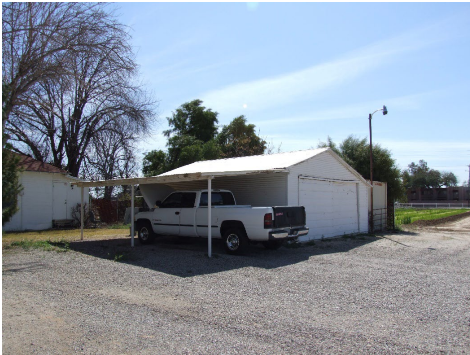
Photograph 3. Overview of the carport at the Residence; view facing southeast (UA_Pima County_UA Campus Agricultural Center Historic District_0003)
