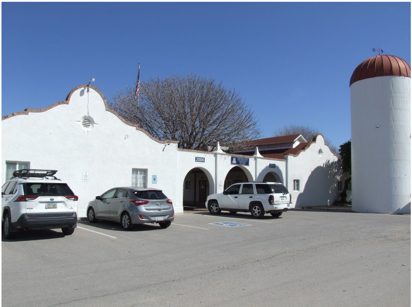
The University of Arizona Campus Agricultural Center, Classroom Building and Office Building, view facing northeast, WestLand Resources, Inc., March 8, 2023.
