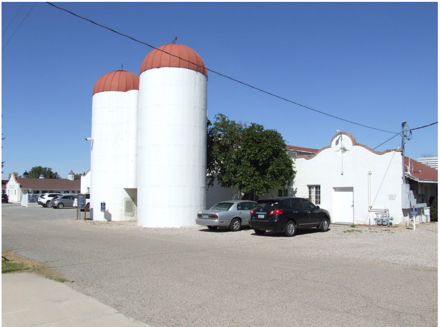
The University of Arizona Campus Agricultural Center, Office Building, view facing northwest, WestLand Resources, Inc., March 8, 2023.
