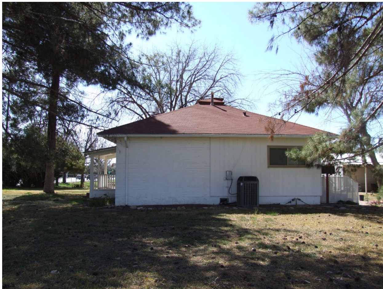
Photograph 4. Overview of north elevation of the Residence; view facing south (UA_Pima County_UA Campus Agricultural Center Historic District_0004)
