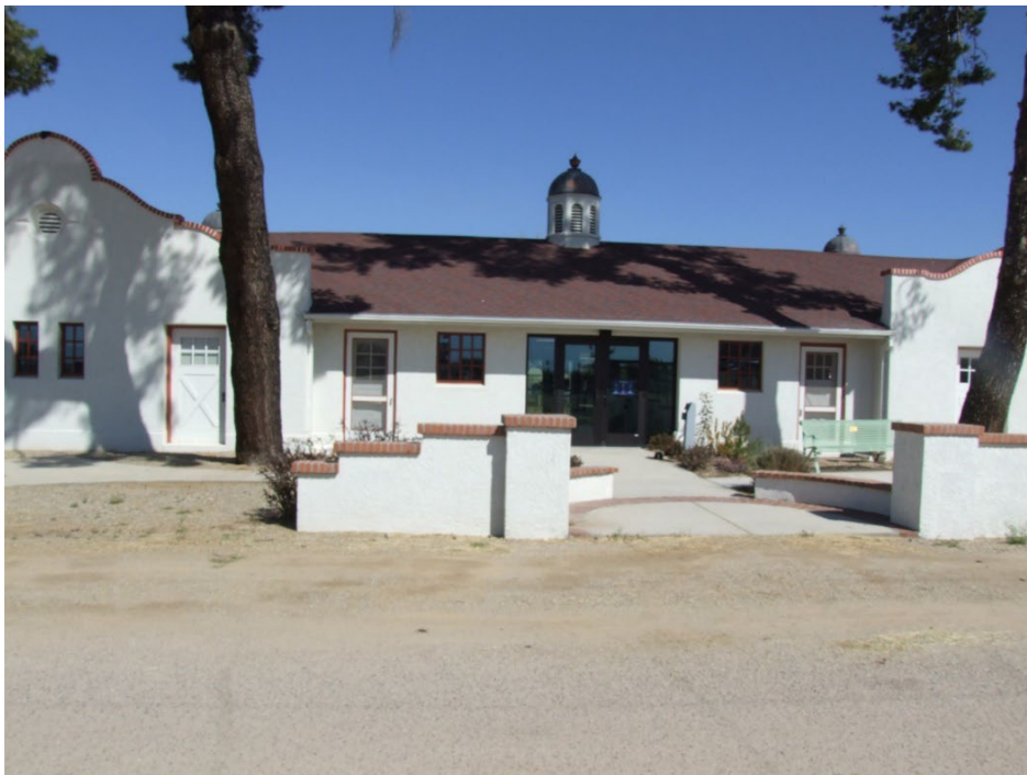
Photograph 20. South elevation overview of the Equine Education Building; view facing north (AZ_Pima County_UA Campus Agricultural Center Historic District_0020)
