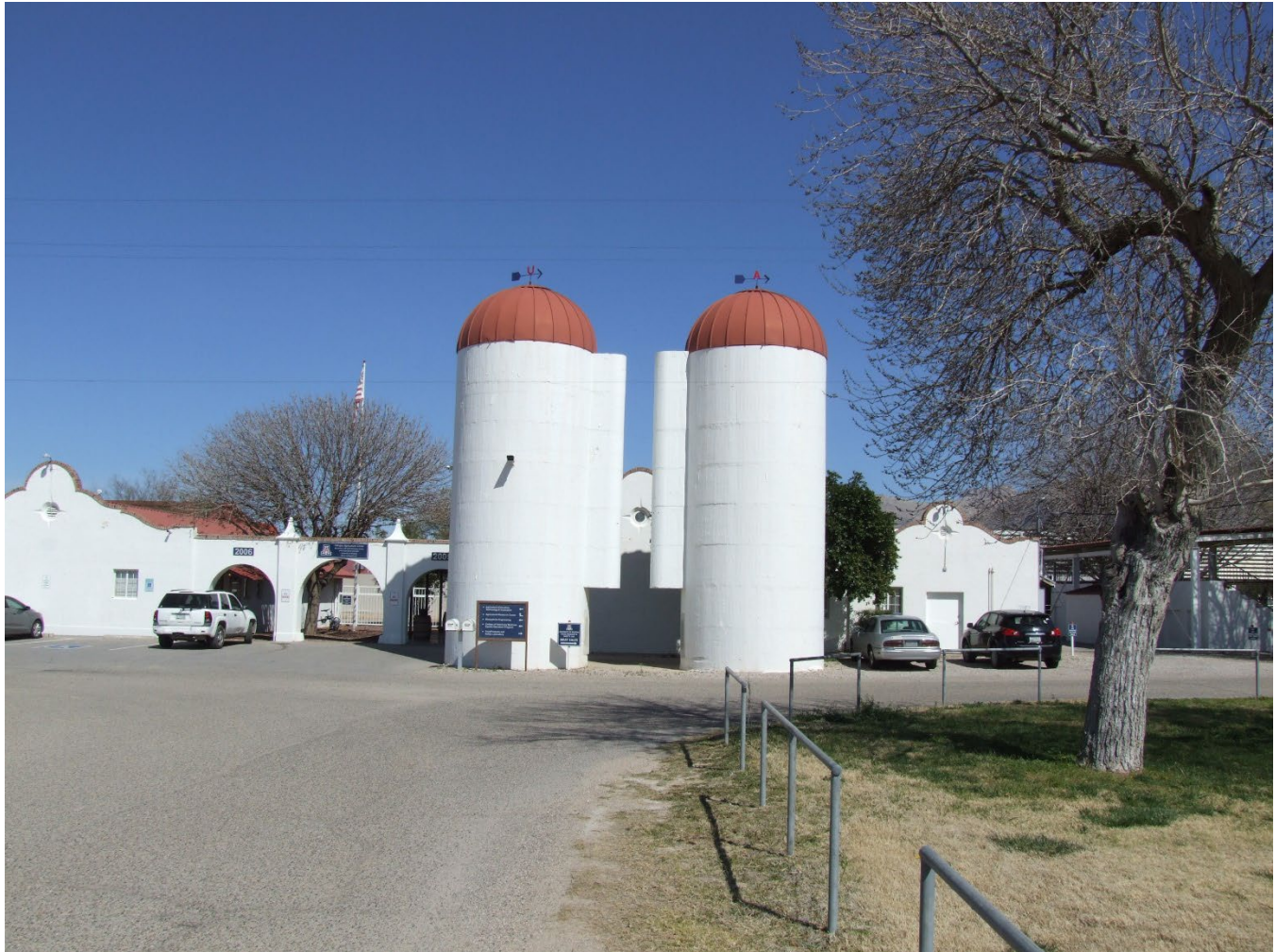
Photograph 15. Overview of south elevations of the two paired silos; view facing north (UA_Pima County_UA Campus Agricultural Center Historic District_0015).
