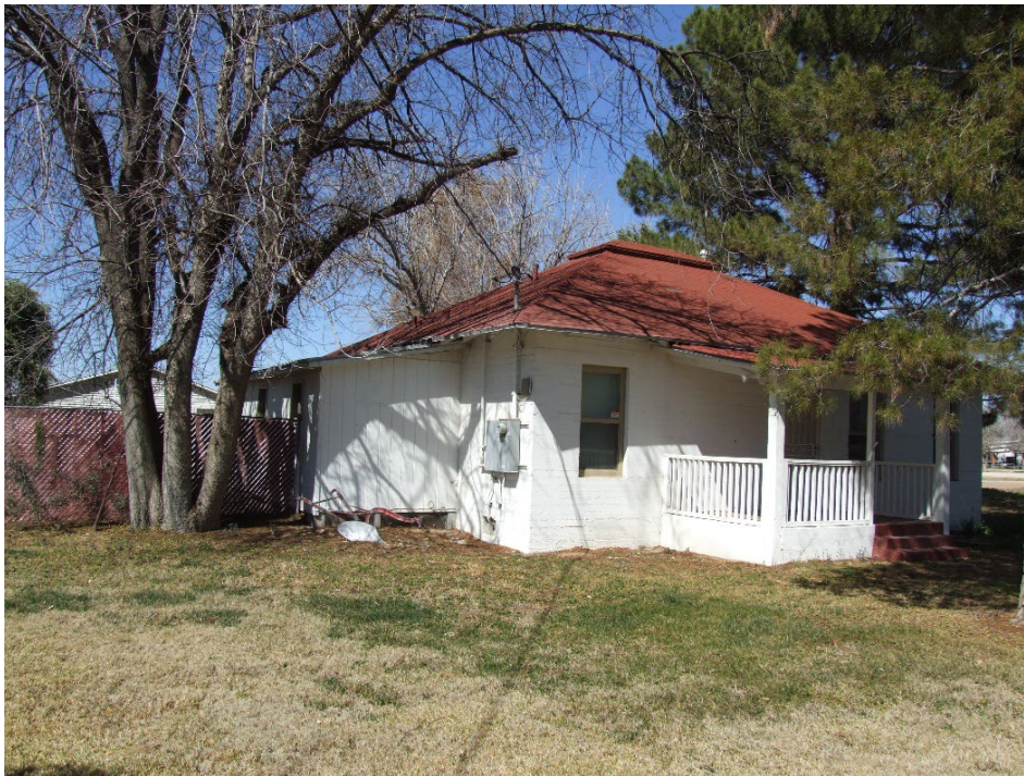
Photograph 6. East and south elevations with south addition of the Residence; view facing northwest (UA_Pima County_UA Campus Agricultural Center Historic District_0006)
