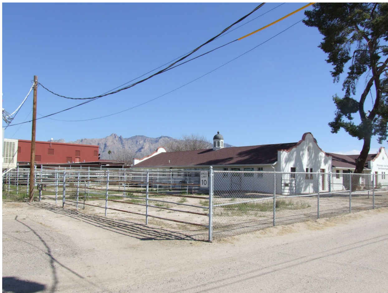
Photograph 13. Overview of Corral and fencing; view facing northeast (AZ_Pima County_UA Campus Agricultural Center Historic District_0013)
