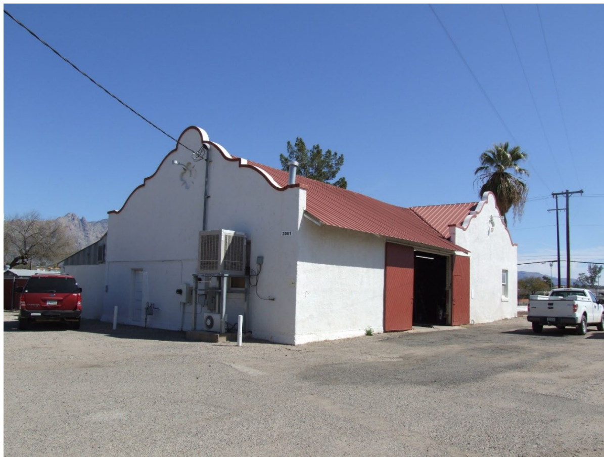
Photograph 9. West and south elevations of the Machine Shop; view facing northeast (AZ_Pima County_UA Campus Agricultural Center Historic District_0009)
