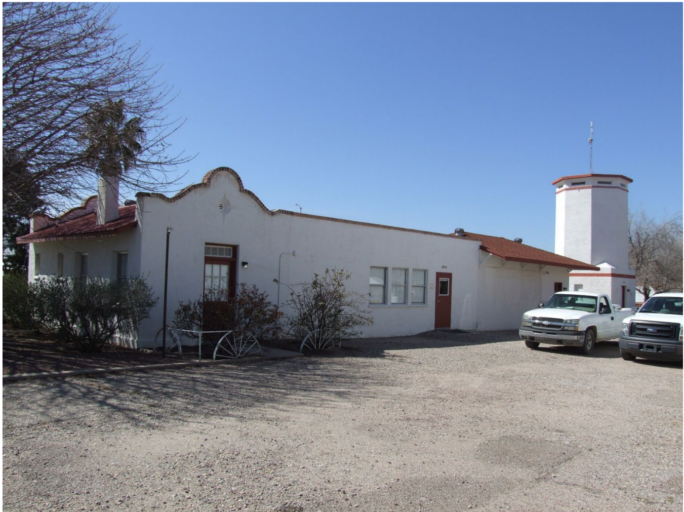
Photograph 23. East and north elevations of the Farm Office; view facing southwest (AZ_Pima County_UA Campus Agricultural Center Historic District_0023).
