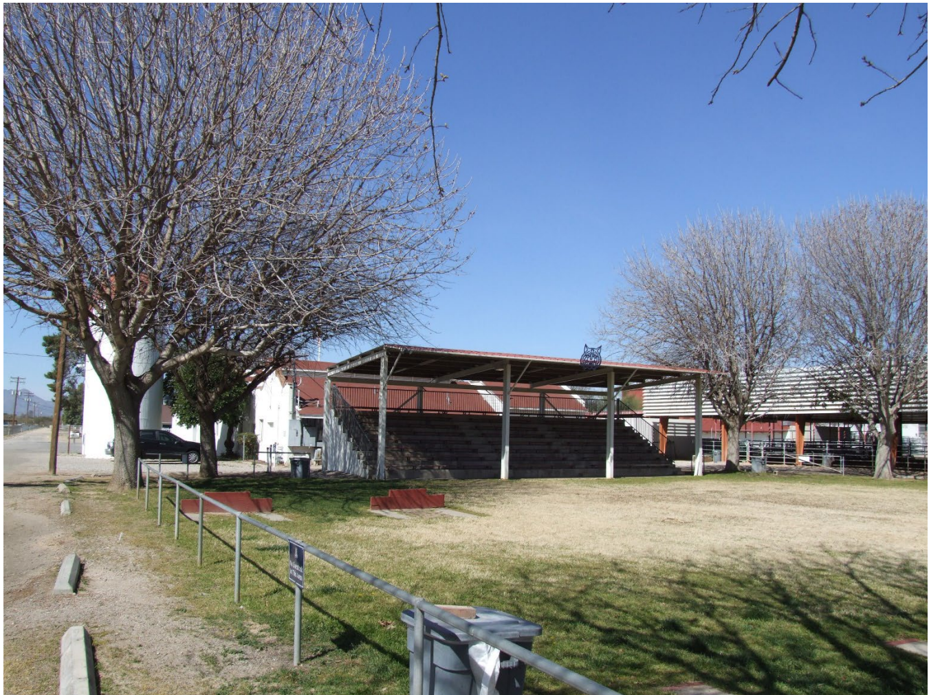
Photograph 26. Overview of Grandstand and field; view facing northwest (AZ_Pima County_UA Campus Agricultural Center Historic District_0026).
