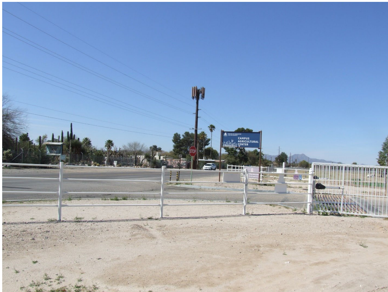
Photograph 25. Overview of original fencing at main entryway and entry signage; view facing west (AZ_Pima County_UA Campus Agricultural Center Historic District_025)
