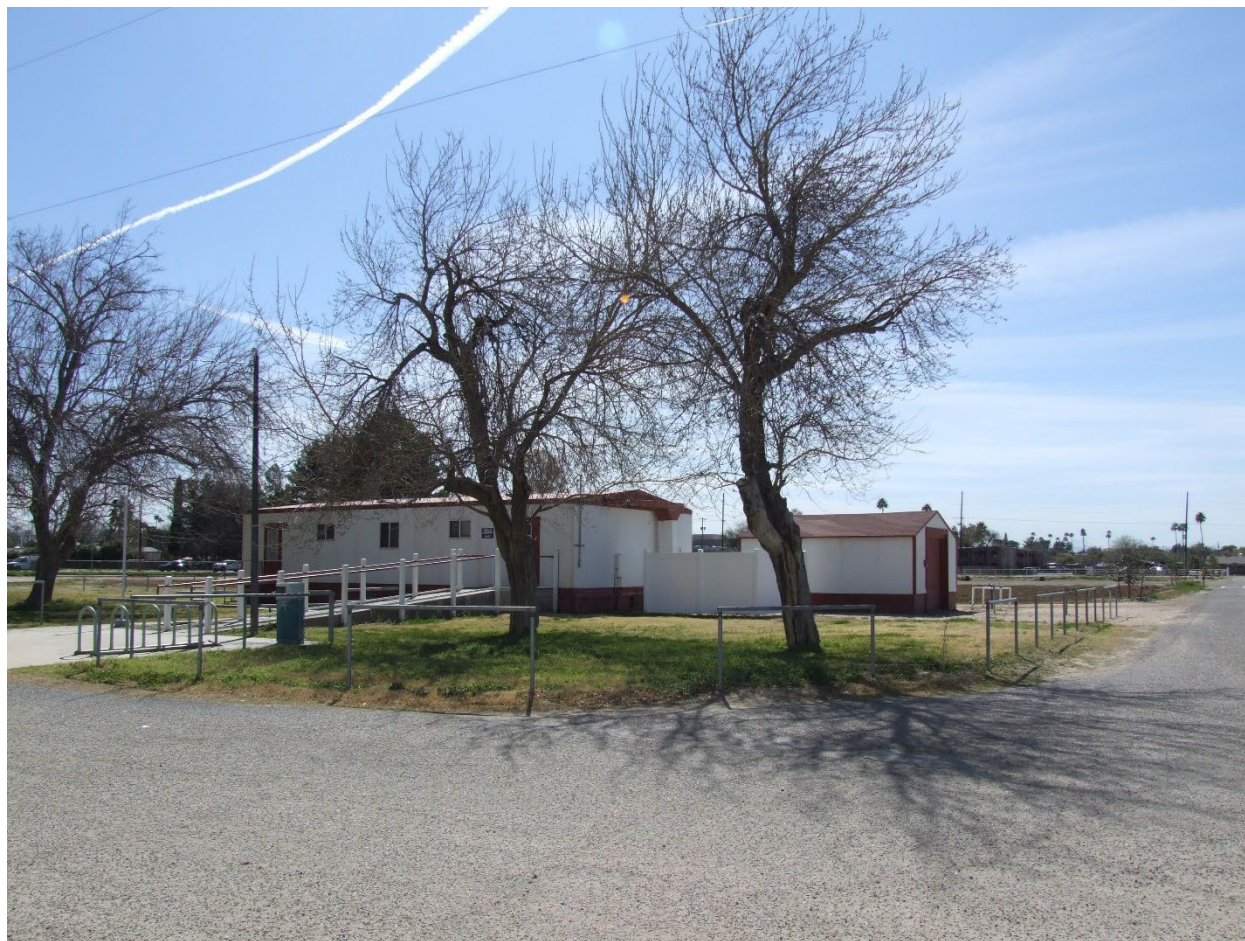
Photograph 28. West and north elevations of the modular Storage building, and storage shed; view facing southeast (UA_Pima County_UA Campus Agricultural Center Historic District_028)
