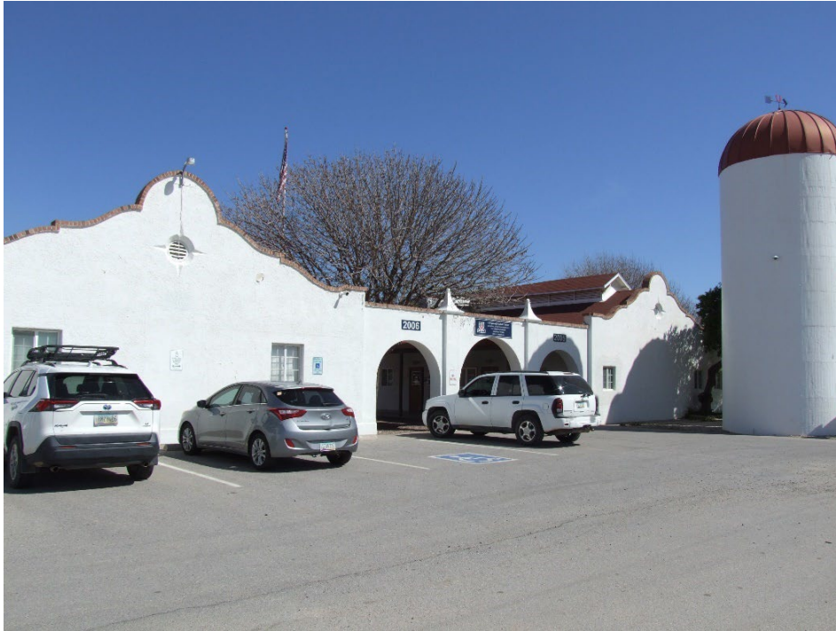
Photograph 16. South elevation of the Office Building and arched arcade openings; view facing northeast (AZ_Pima County_UA Campus Agricultural Center Historic District_0016)
