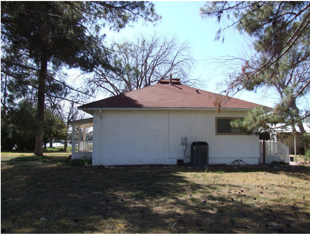
The University of Arizona Campus Agricultural Center, Main Residence, north elevation, view facing south. WestLand Resources, Inc., March 8, 2023.
