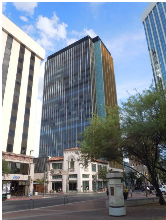
Photo 8: AZ_Pima_DowntownTucsonHistoricDistrict_0008 (August 2012) Tucson Federal Savings (32 N. Stone Ave.) (center) north façade (left) and west façade (right), camera facing southeast
