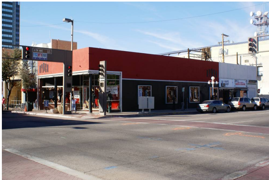
Photo 7: AZ_Pima_DowntownTucsonHistoricDistrict_0007 (January 2012) Dave Bloom and Sons (145 E. Congress St.), south façade (left) and east façade (right), camera facing northwest
