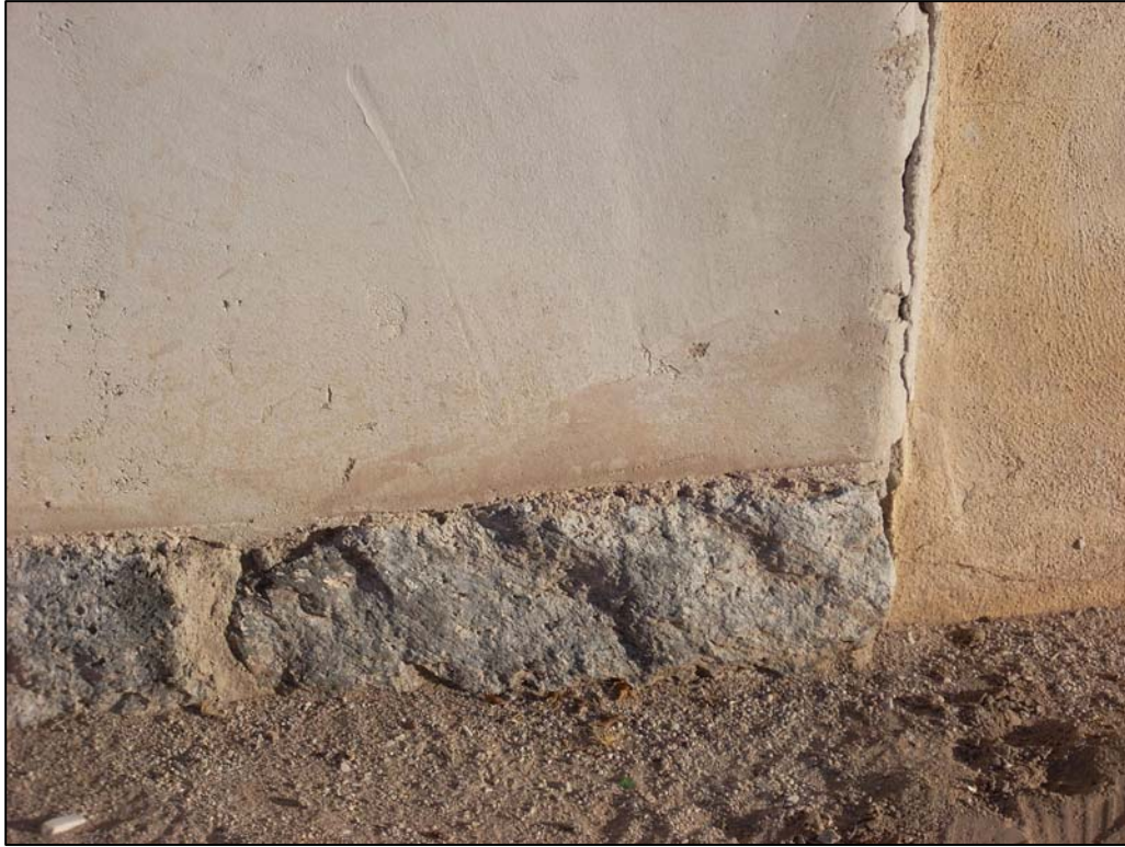
Photo 10. Detail of shaped boulder foundation of the adobe at 738/612 S. 8th Avenue.
