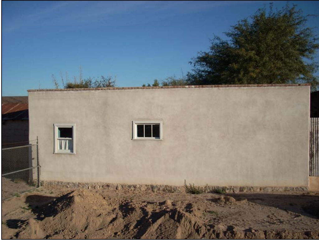
Photo 5. Adobe structure at 738/612 S. 8th Avenue; view to the north.
