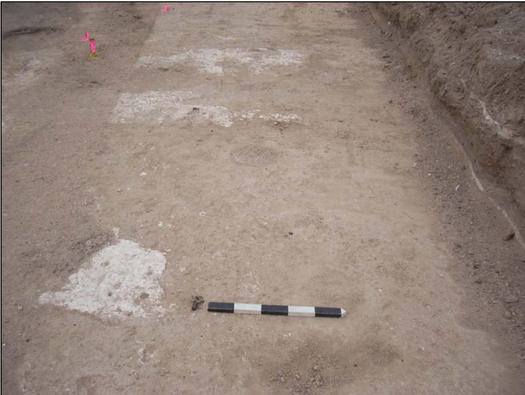
Photo 40. Possible concrete foundation footprint in Feature 4, north side of BHT 3.
