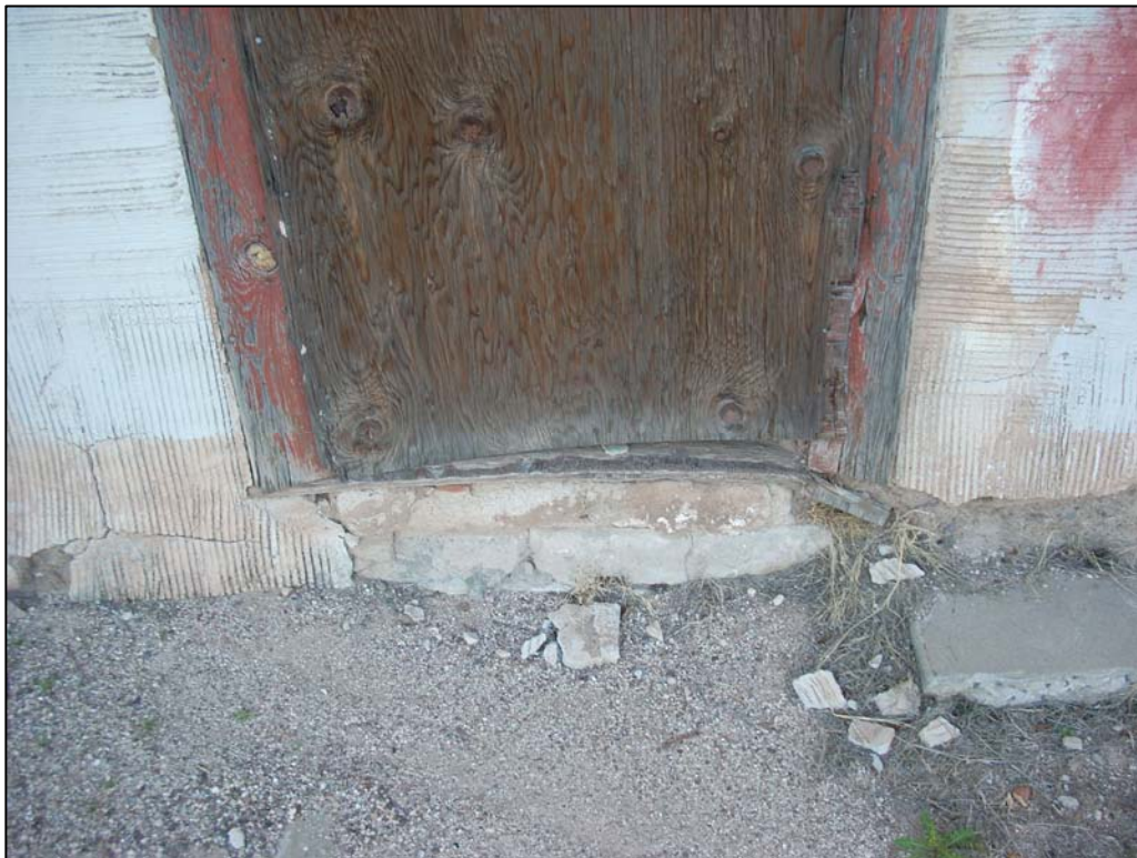
Photo 13. Detail of elevated brick/lumber threshold of the doorway at the southern end of the house at 576 S. 8th Avenue.
