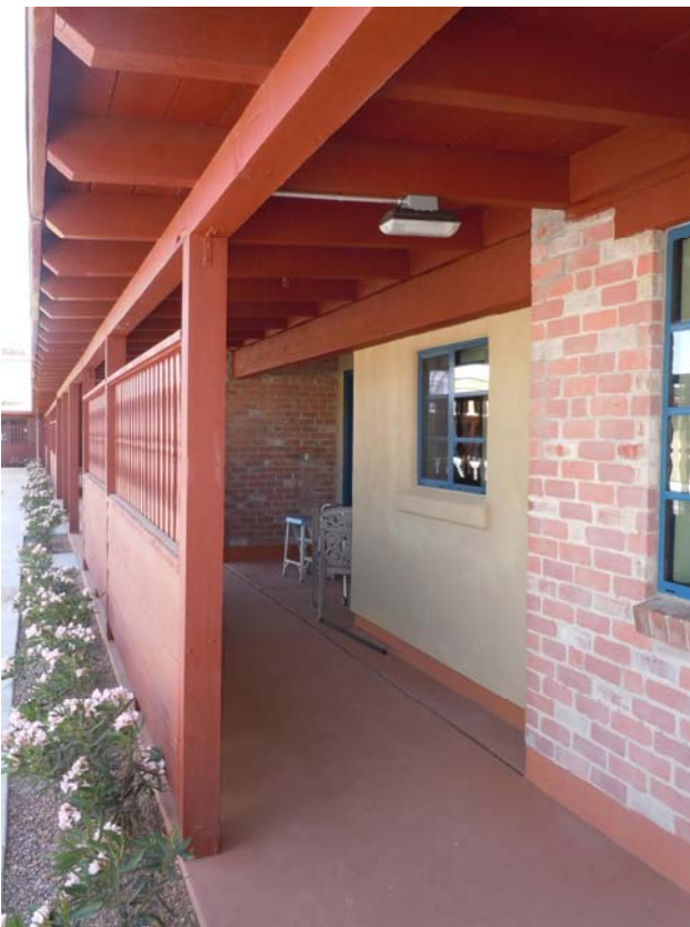
20. First Building Group Addition Building K carport infill retains sense of space and original grilles. View to south. (Photo by Don W. Ryden of Ryden Architects, Inc., 2011)
