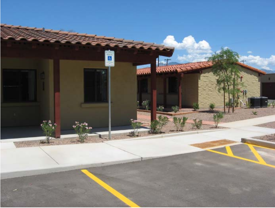
32. Fourth Building Group Addition The simple details and finishes of the new Apartment (Building 4) (foreground) defer to and complement the historic character of the Joesler-designed Building D (background). View to northeast. (Photog by Don W. Ryden of Ryden Architects, Inc., 2011)
