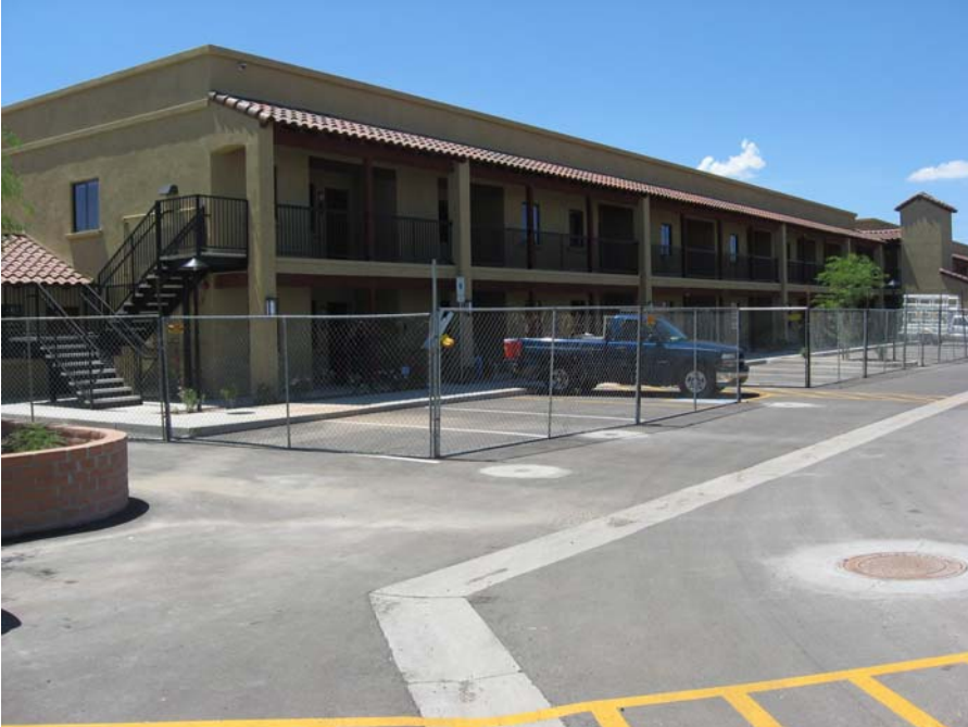
33. Fourth Building Group Addition The new, two-story Apartment (Building 5) stands at the rear of the property where its height has no adverse effect on the one-story historic buildings. View to southwest. (Photo by Paul C. Sikorski of Ryden Architects, Inc., 2010)
