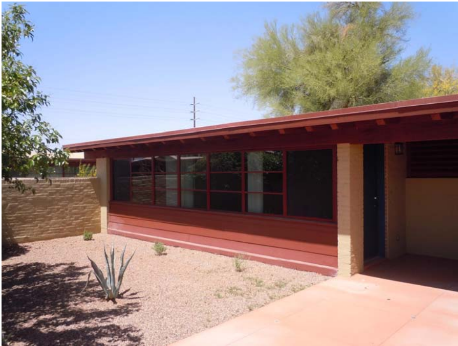
24. Second Building Group Addition Contemporary Style duplex (Building O) with original walled patio area. View to northwest. (Photo by Don W. Ryden of Ryden Architects, Inc., 2011)
