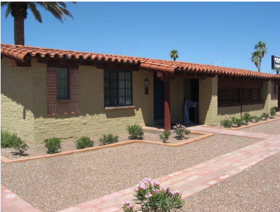
16. Original Building Group Joesler-designed Spanish Colonial Revival casita (Building E) with private porch and carport. View to northwest. (Photo by Paul C. Sikorski of Ryden Architects, Inc., 2010)
