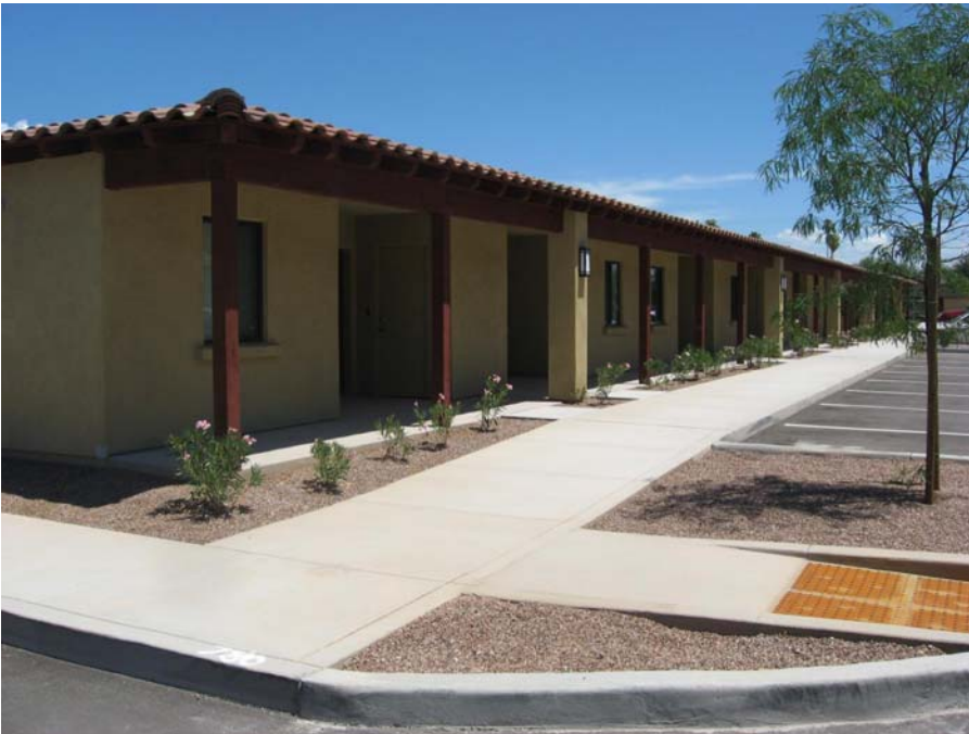
31. Fourth Building Group Addition The new, one-story Apartment (Building 4) is a simplified interpretation of the Joesler-designed duplexes. View to northeast. (Photo by Don W. Ryden of Ryden Architects, Inc., 2011)
