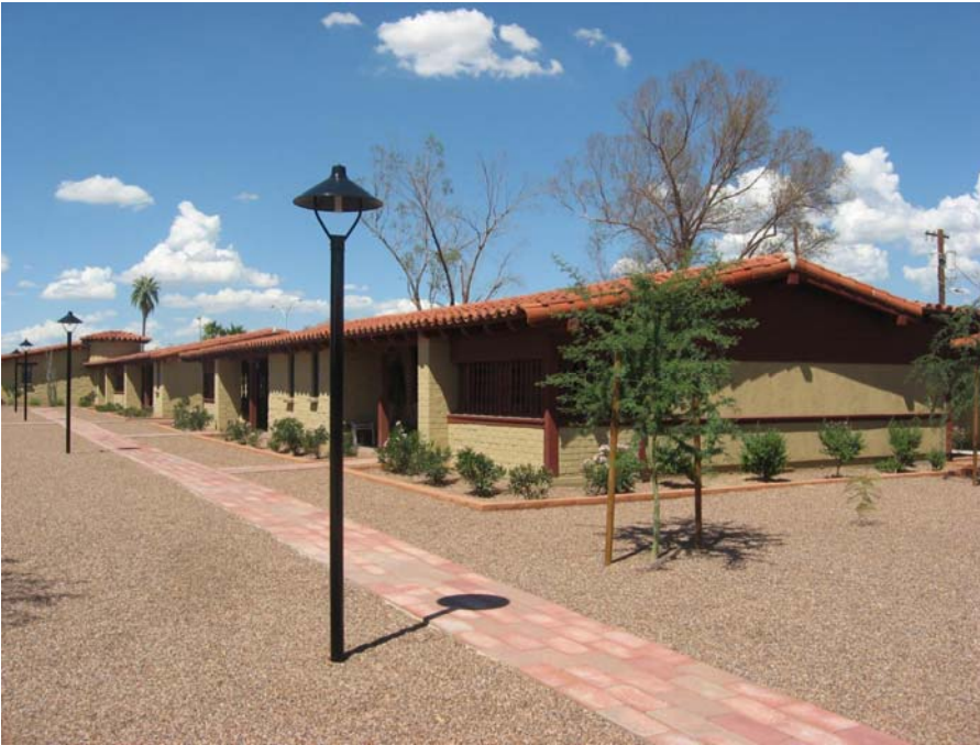
9. Original Building Group Building D and C. View to northeast. (Photo by Paul C. Sikorski of Ryden Architects, Inc., 2010)
