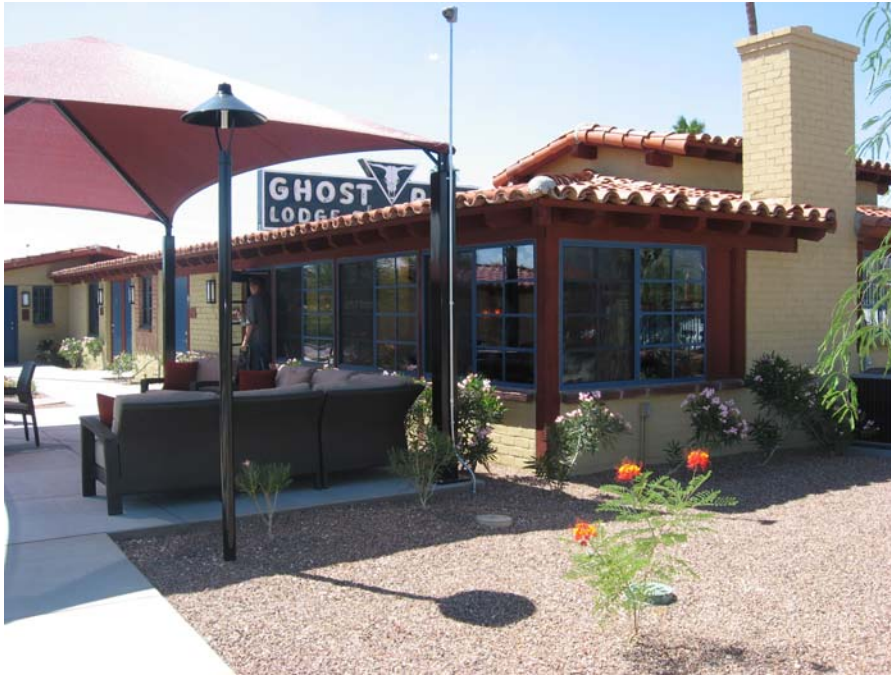
7. Original Building Group South patio behind rehabilitated Office Q. View to northwest. (Photo by Paul C. Sikorski of Ryden Architects, Inc., 2010)
