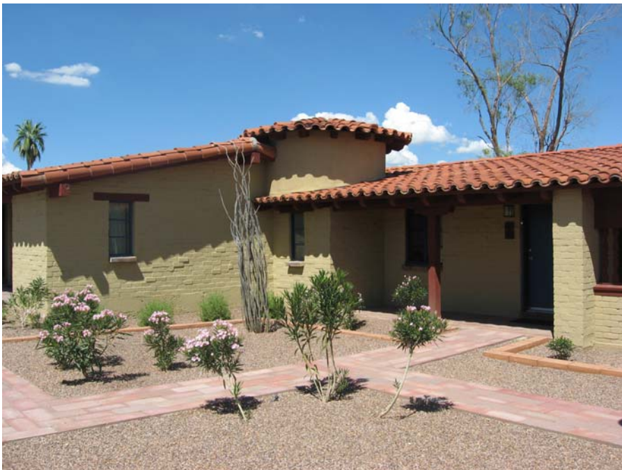
8. Original Building Group Rehabilitated porch and tower at Building D. View to northeast. (Photo by Don W. Ryden of Ryden Architects, Inc., 2011)
