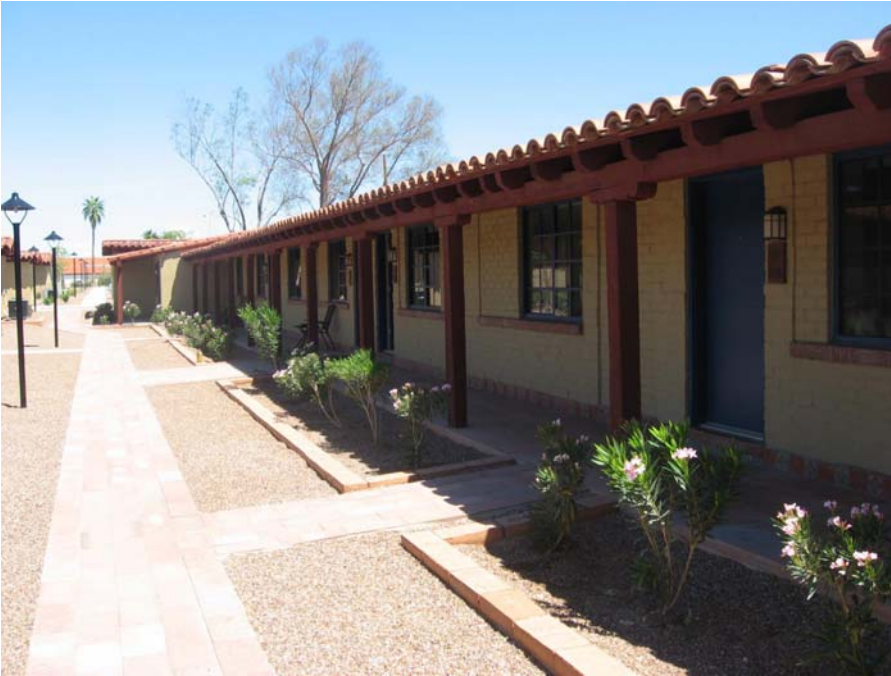
17. First Building Group Addition Spanish Colonial Ranch Style linear units (Building A) with coverd walkway and no carports. View to northeast. (Photo by Paul C. Sikorski of Ryden Architects, Inc., 2010)
