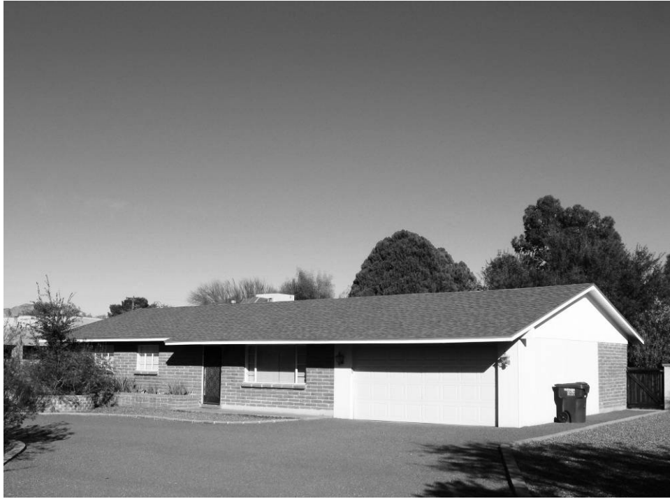
Figure 30. 920 N. Wilmot Rd.; view northeast.
