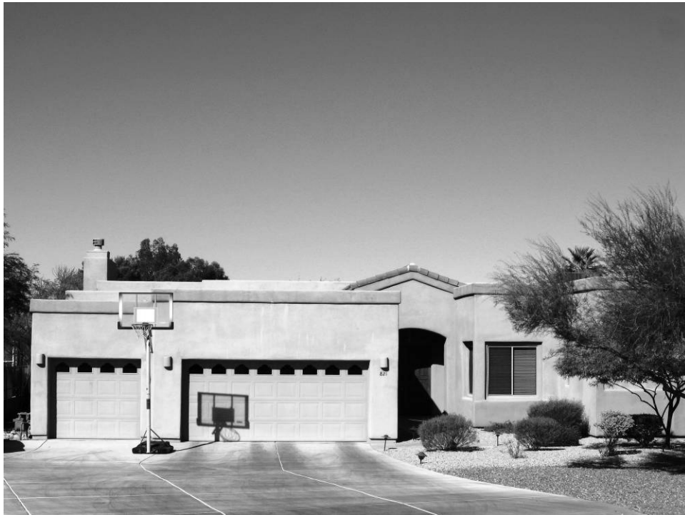
Figure 29. 821 N. Barbara Worth Dr.; view west-northwest.
