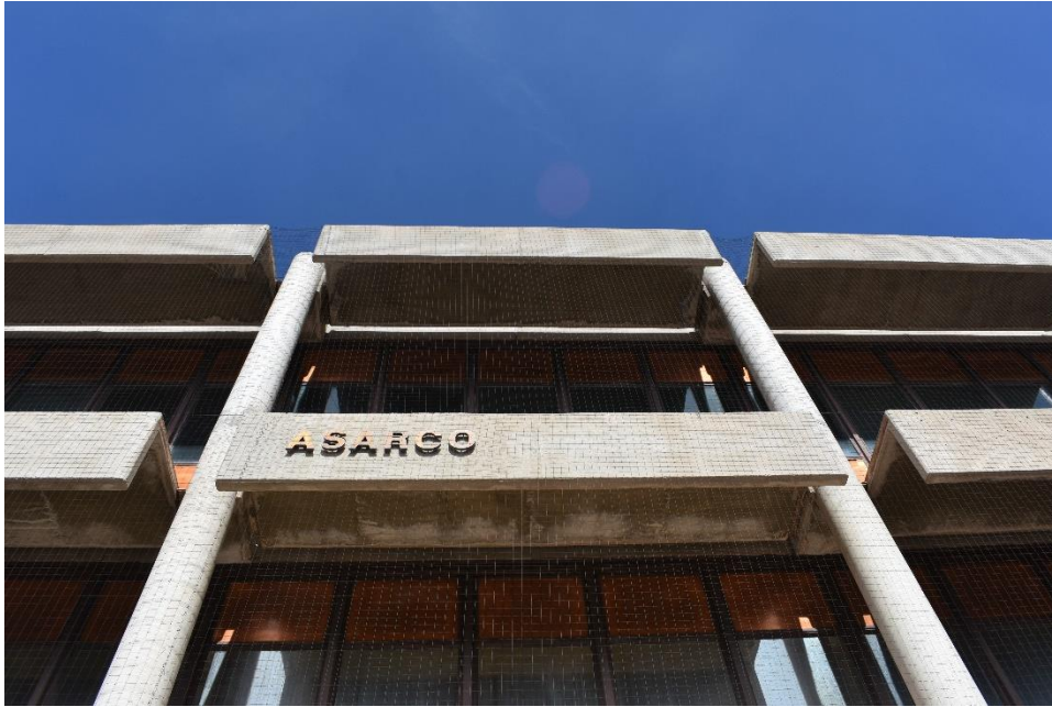
Figure 5. ASARCO Headquarters, showing south elevation, looking up (Logan Simpson 2021 [AZ_PimaCounty_ASARCOHeadquarters_0003]).
