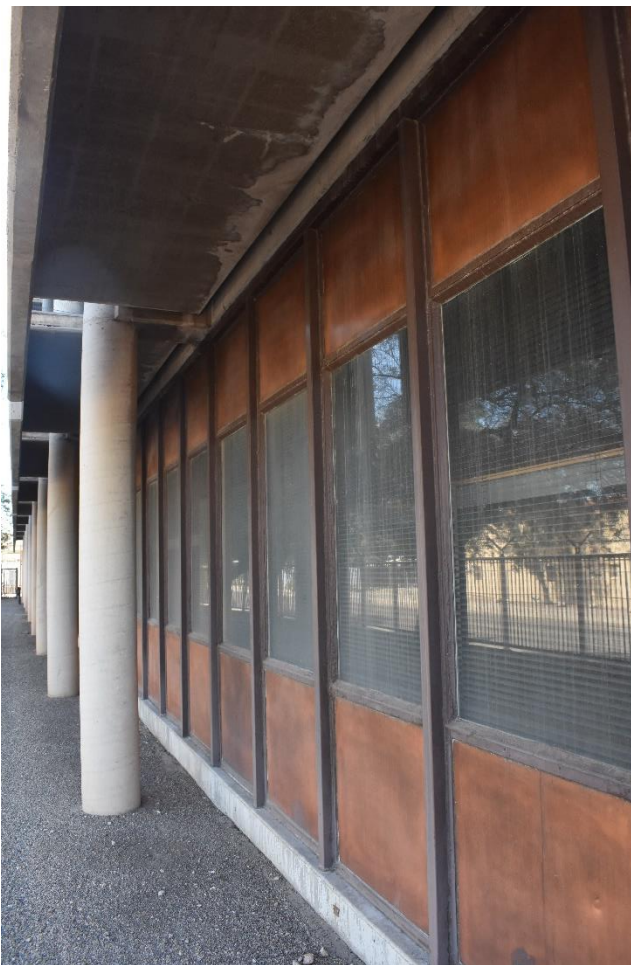
Figure 6. ASARCO Headquarters, facing northwest (Logan Simpson 2021 [AZ_PimaCounty_ASARCOHeadquarters_0004]).
