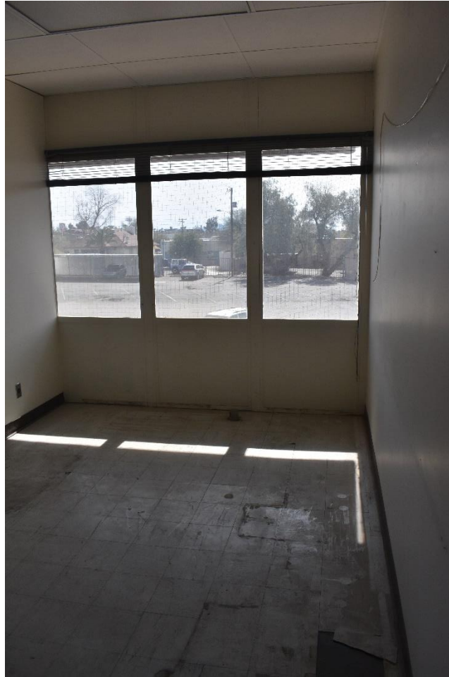
Figure 13. ASARCO Headquarters, showing first story from lobby, looking east (Logan Simpson 2021 [AZ_PimaCounty_ASARCOHeadquarters_0011]).
