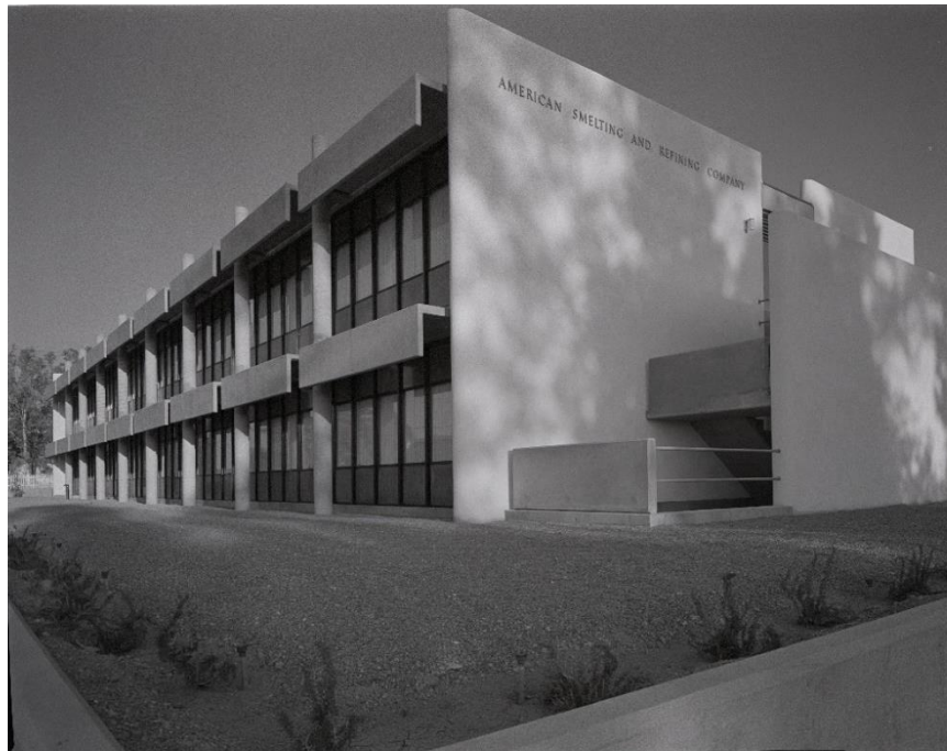
Figure 24. ASARCO Headquarters building as originally constructed showing solid end massing with recessed sides. Note the exposed tops of the columns which are poised for continued upward expansion. Looking southeast c. 1965. (Courtesy of the Tucson Historic Preservation Foundation, Bill Sears Collection)
