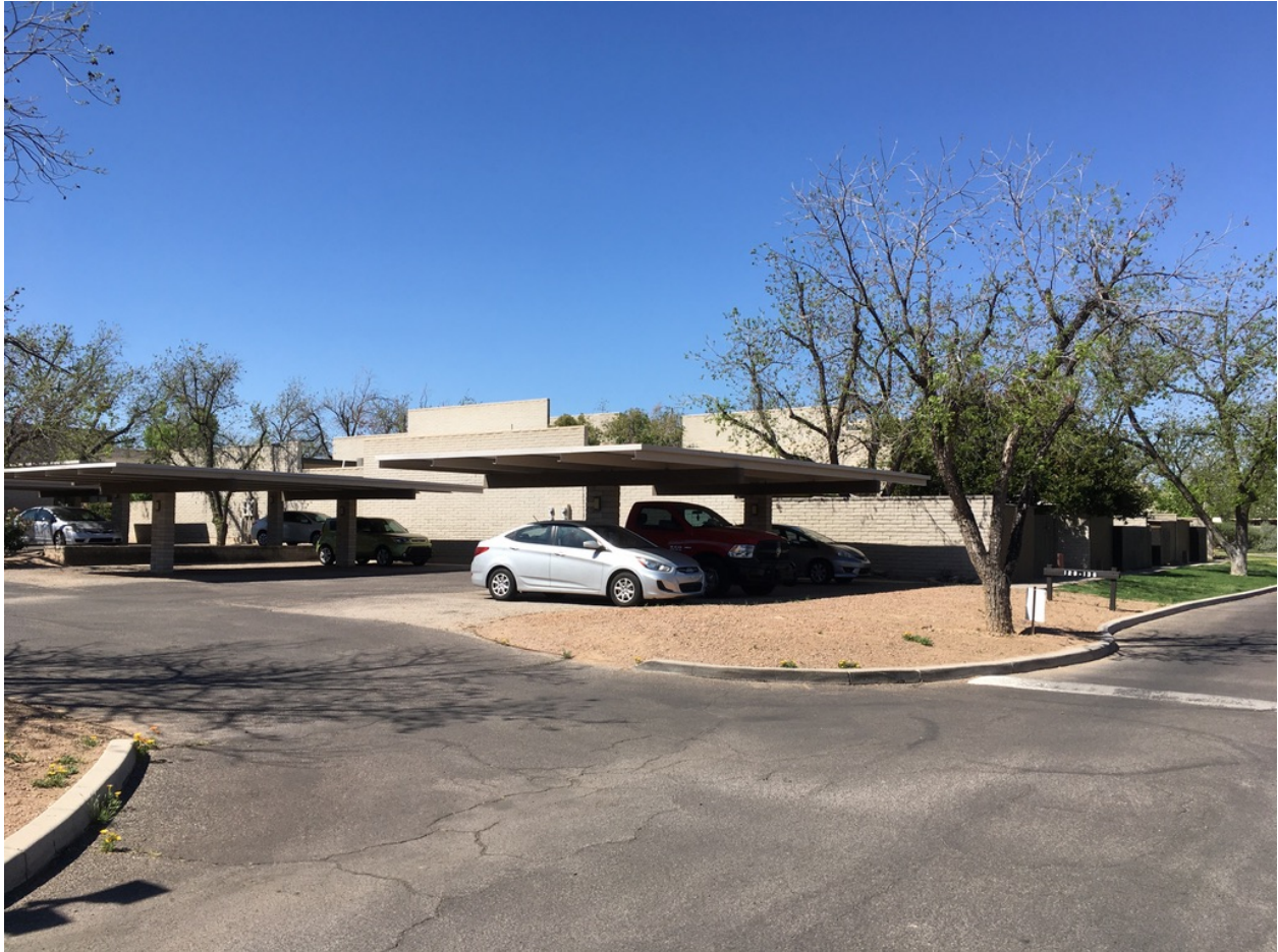
Photo 16: View of parking ramadas, planar walls and pecan trees, looking southwest. 2021
