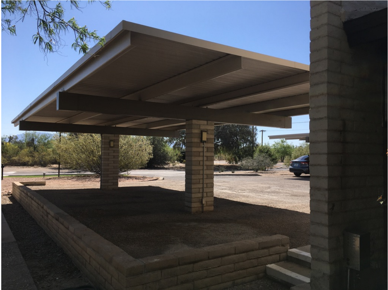
Photo 40: Close up view of one of the parking ramadas. 2021
