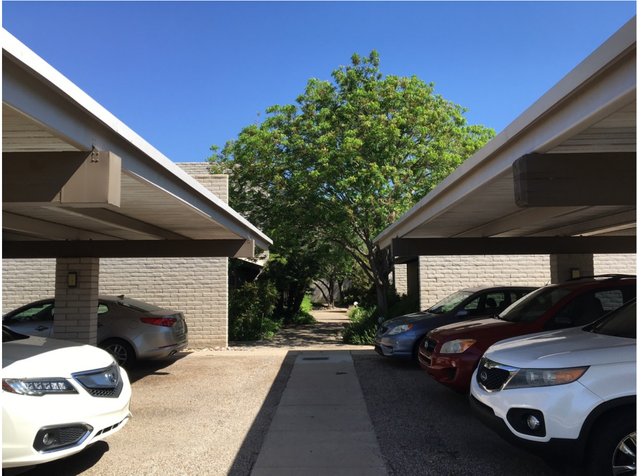
Photo 31: View into entry courtyard from parking area, looking north. 2021
