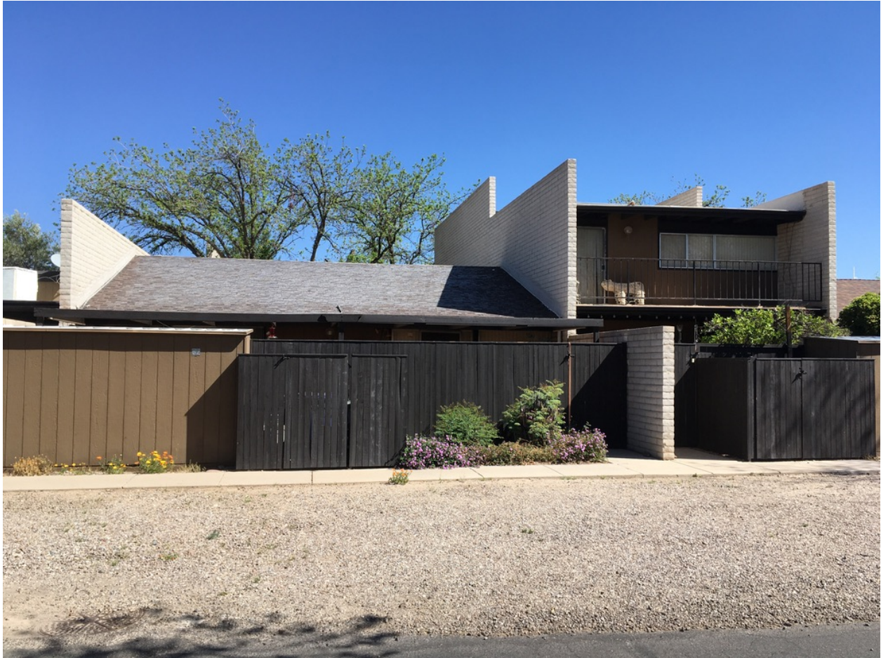
Photo 11: View of back (patio) side of townhomes from primary driveway, looking north. 2021
