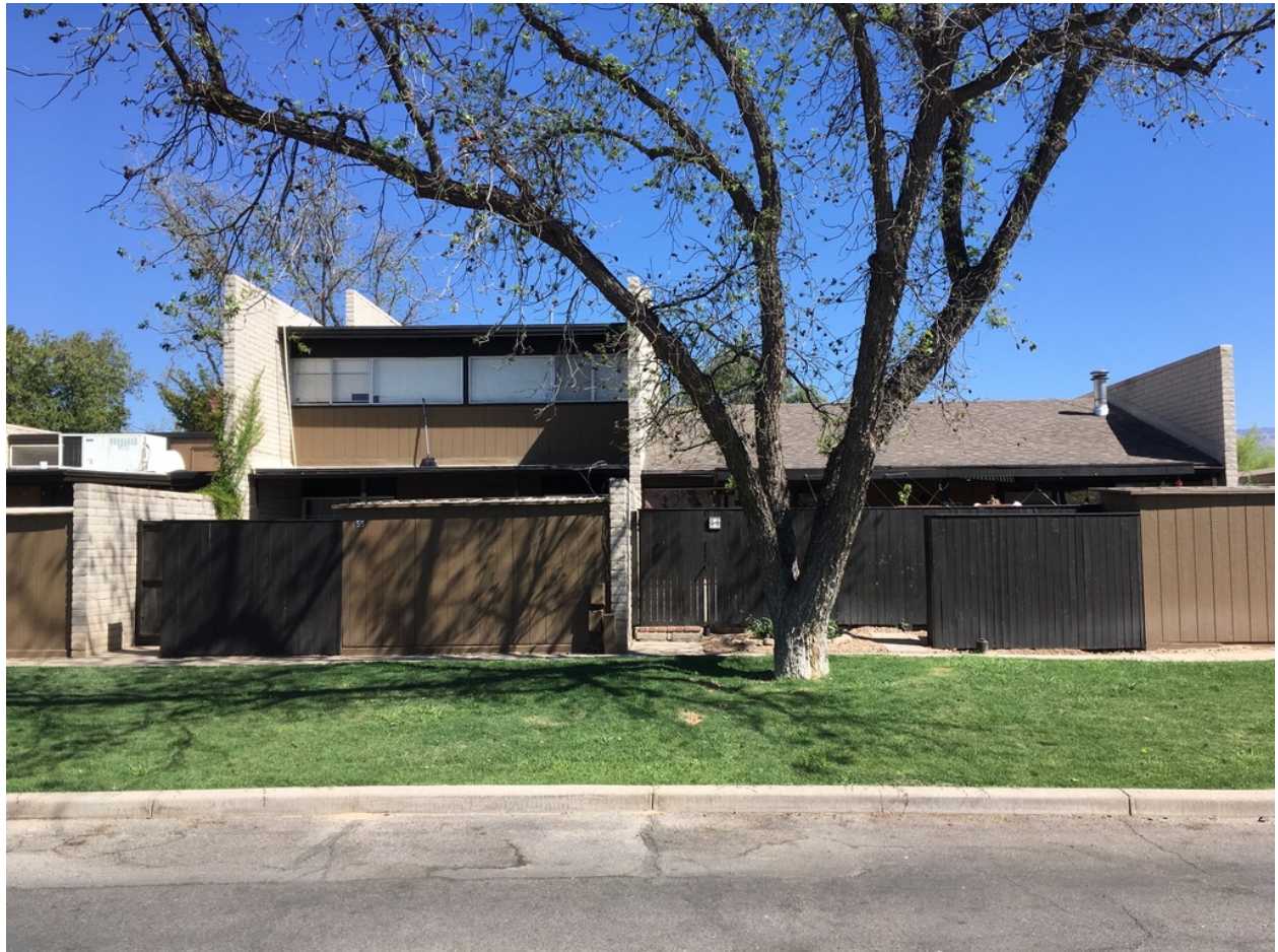
Photo 14: View of back (patio) side of townhomes from primary driveway, looking north. 2021
