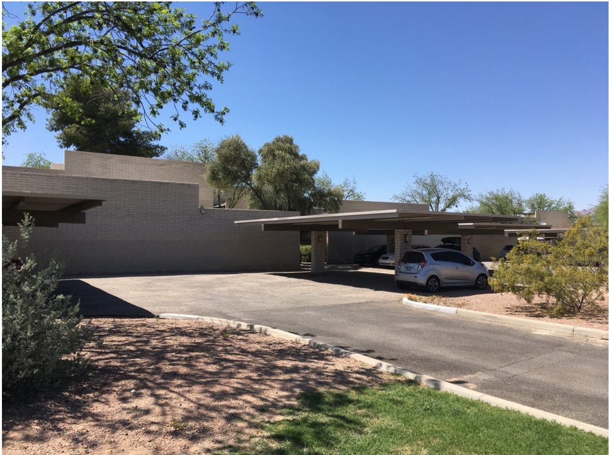
Photo 8: View of parking area, planar walls, and entry into one of the courtyards, looking northwest. 2021
