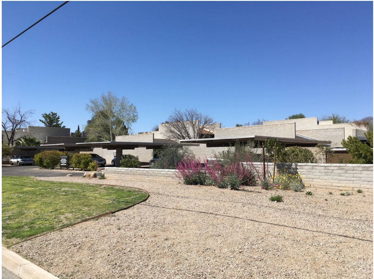
Photo 44: Winter view showing the layered character of the planar masonry walls. 2021
