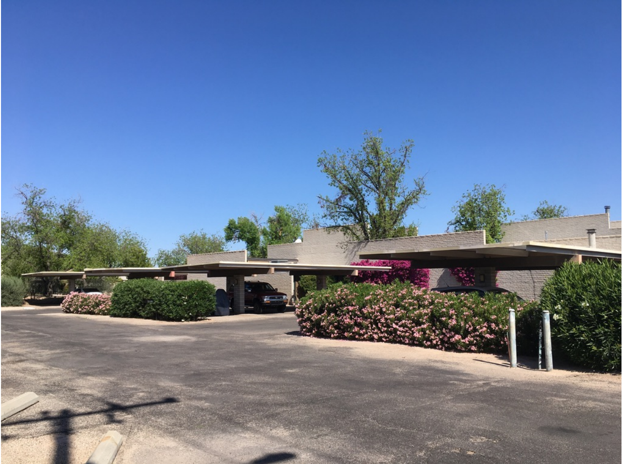
Photo 5: View of parking ramadas and planar walls from Glenn St. 2021
