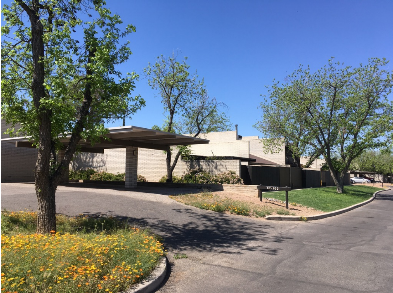
Photo 13: View along primary driveway, looking southwest. 2021
