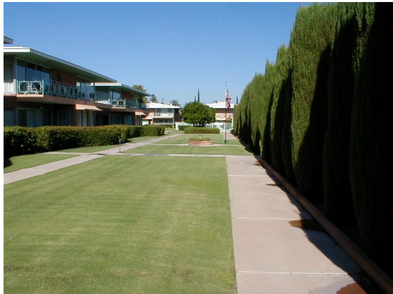
Fig. 12: Villa Catalina Apartments courtyard
