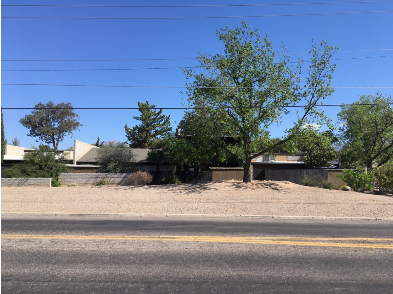
Photo 6: View of back (patio) of townhomes from Glenn St. 2021
