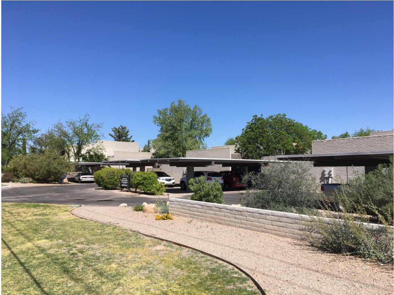
Photo 7: View of parking ramadas and planar walls from Glenn St. 2021
