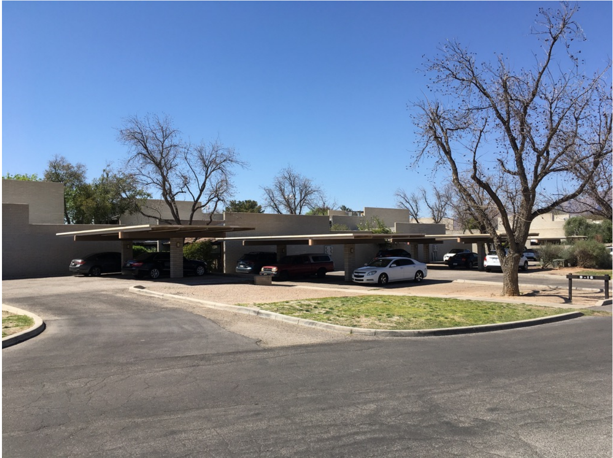
Photo 43: Winter view showing the layered character of the planar masonry walls. 2021
