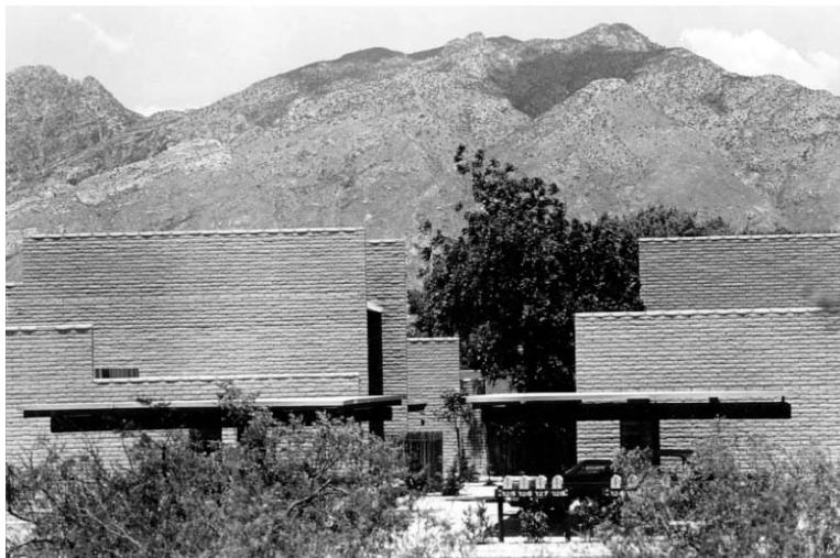
Fig. 9: Historic photo (early 1970s) from south side of Glenn St., looking north
