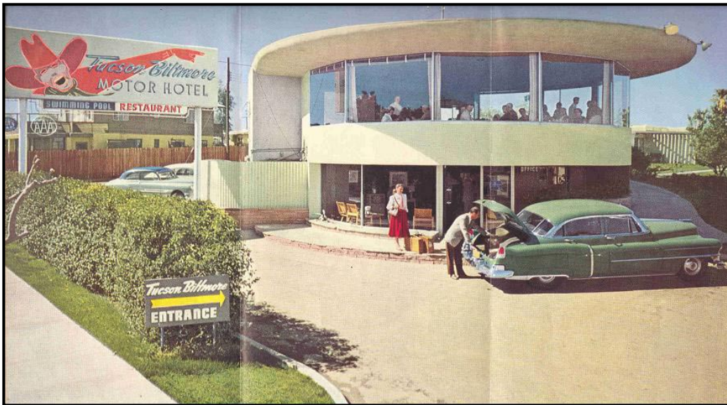
Tucson Biltmore Motor Hotel, advertising brochure. ca. 1960. (Demolished) (Courtesy Dirk Arnold)
