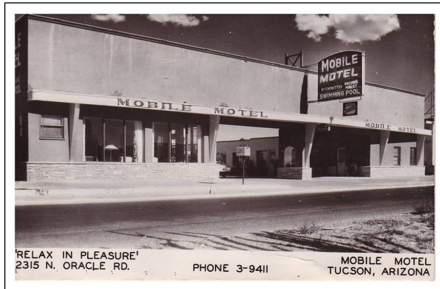
Mobile Motel, Oracle Road ca 1950. (demolished) (Courtesy Tucson Post Card Club)
