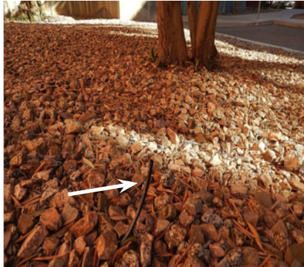
This micro-tube delivers water to the root zone of the tree. Under ground, it is attached to an emitter connected to a polyethylene tube.
