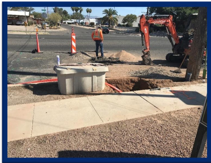
Figure 12: Pullbox prior to installation
