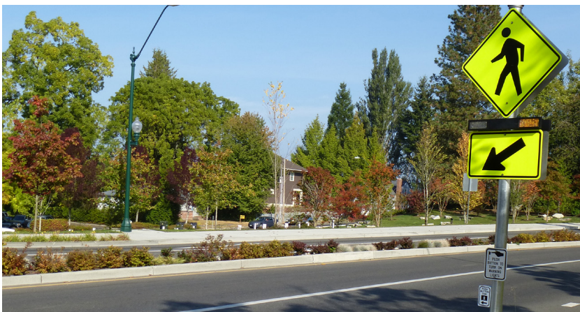
Image 5.4 RRFBs improve driver compliance at crossings. Credit: Toole Design Group
