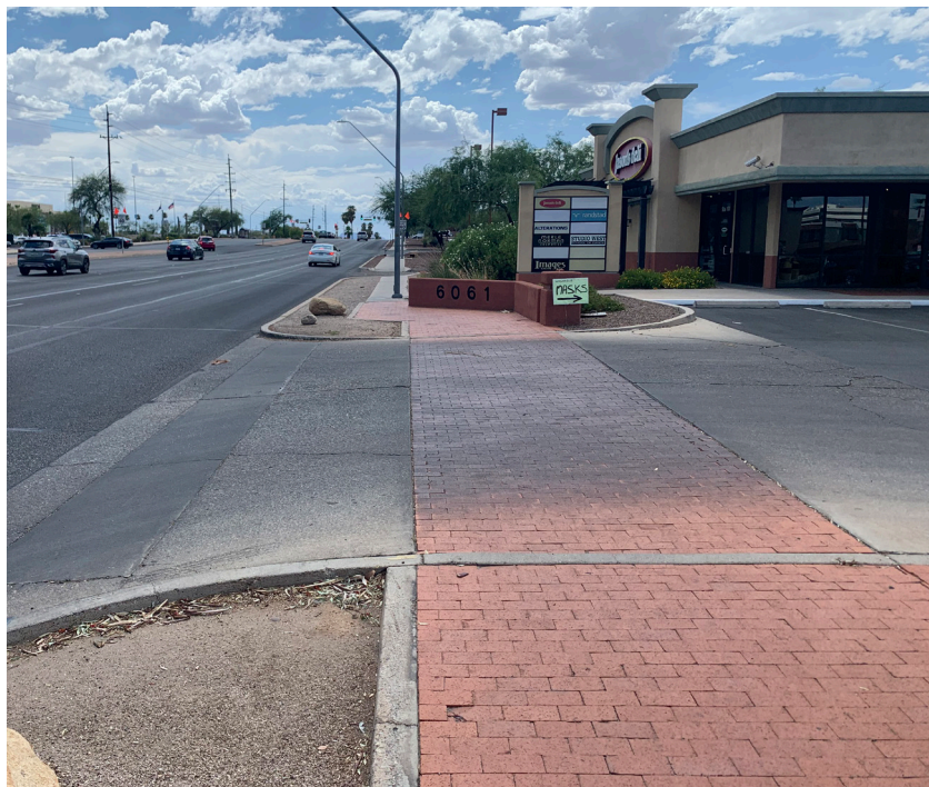
Image 3.8 Level sidewalk crossing at driveway with sidewalk dominant
