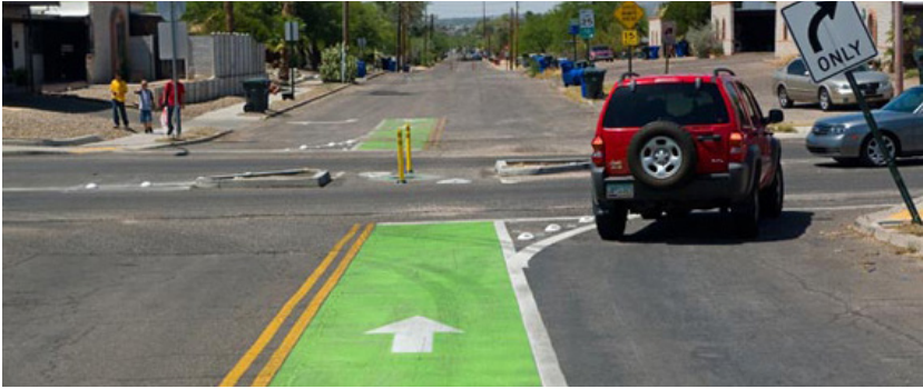
Image 4.30 A Median Barrier with Forced Turn Island
