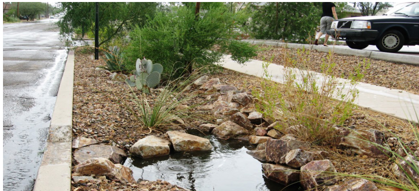
Image 6.6 Green infrastructure basin behind curb Credit: Watershed Management Group
