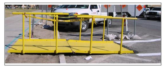
Use of pedestrian bridges requires that a 4"X 4' level landing area be provided at both ends of the ramp.
