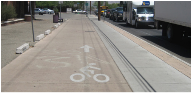
Cyclists using the Third Street Bicycle Boulevard are directed along a two-way separated bike path adjacent to the sidewalk in order to make the offset crossing at Alvernon Way.
