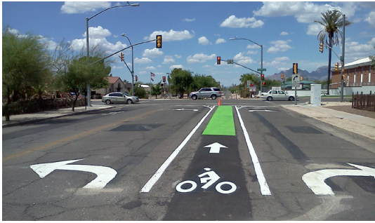
Right- and left-only turns restrict cut through traffic along Fourth Avenue at Speedway Boulevard.
