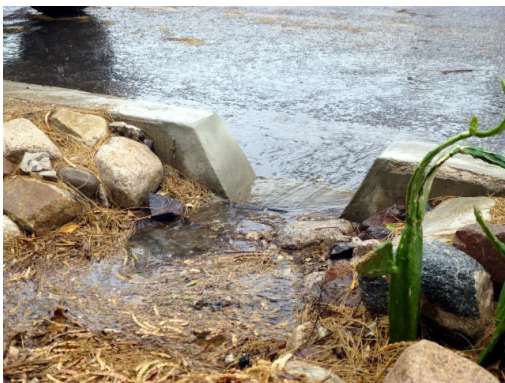
Curb cuts allow stormwater runoff to enter a landscaped basin in the public right of way (Photo credit: Watershed Management Group)
