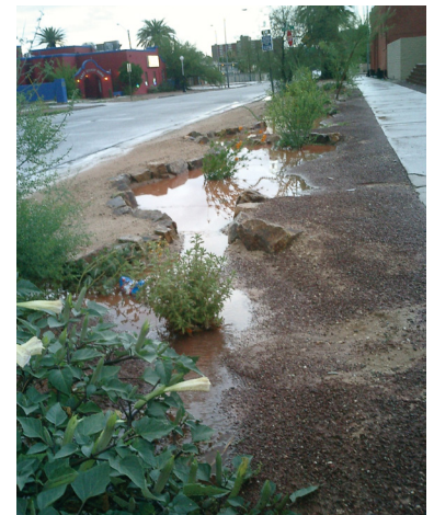
A landscaped basin along Park Avenue captures water during a storm (Photo credit: Watershed Management Group)
