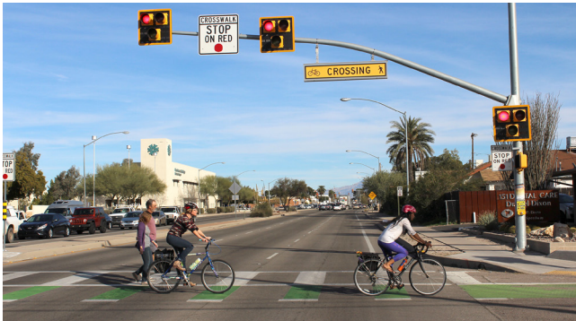
Pedestrian and cyclists cross Speedway Boulevard at a BikeHAWK on 10th Avenue.
