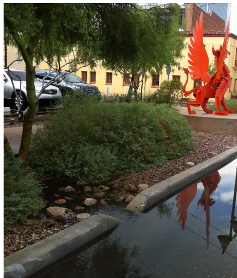
Stormwater infiltrates a catchment basin with native landscaping along Scott Avenue (Photo credit: Watershed Management Group)
