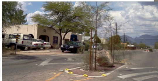
Combined speed hump with landscaped center median
