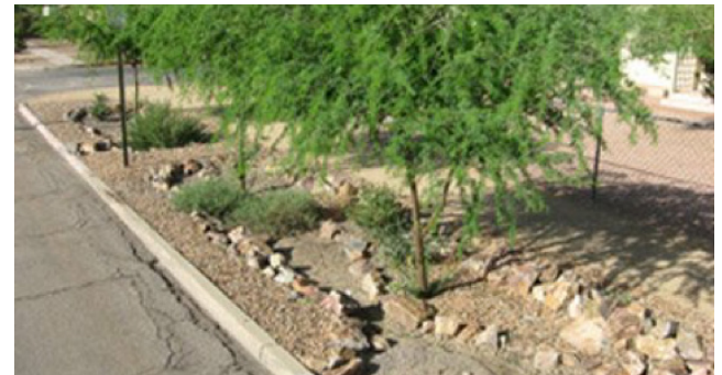
A curb cut and bioswale captures stormwater while native trees provide shade for cyclists and pedestrians.
