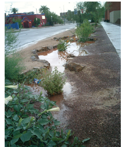
A landscaped basin along Park Avenue captures water during a storm (Photo credit: Watershed Management Group)
