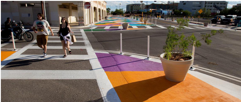
Image 4.33 Demonstration public plaza and curb extensions on 6th Ave and 7th St in Tucson
