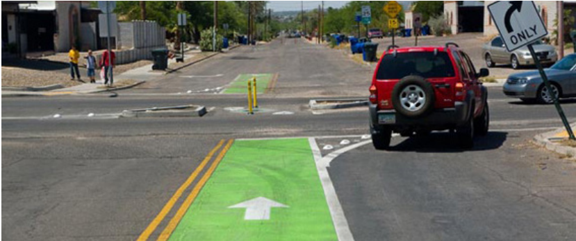
Image 4.30 A Median Barrier with Forced Turn Island
