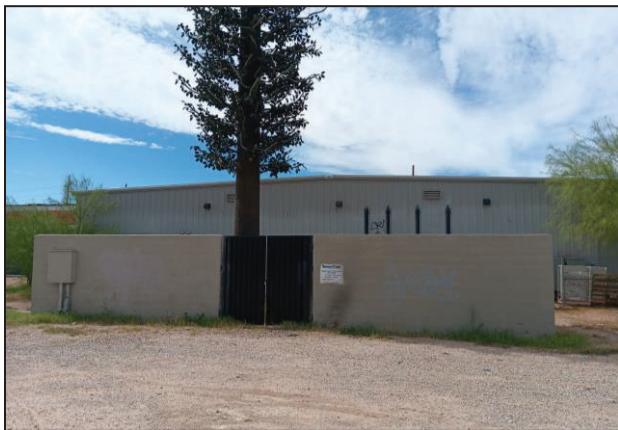
Picture 3 – View of cell tower on the Subject Property
