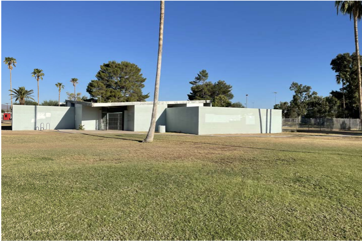
Project south elevation, poolhouse, bath/showers, storage, offices (facing north)
