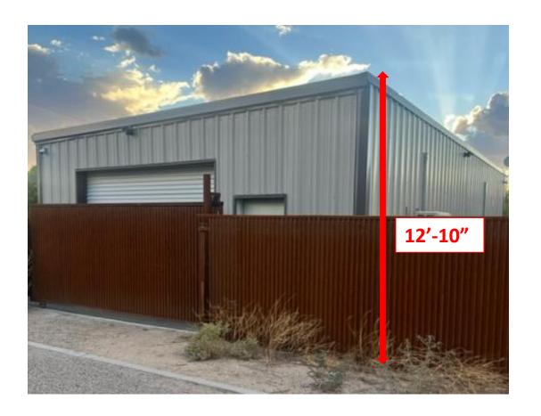
Item 2: Article 6.4.4.A Measurement of Building Height, defines the building height as the vertical distance measured from the design grade elevation to the middle of the highest gable of a pitched roof.
