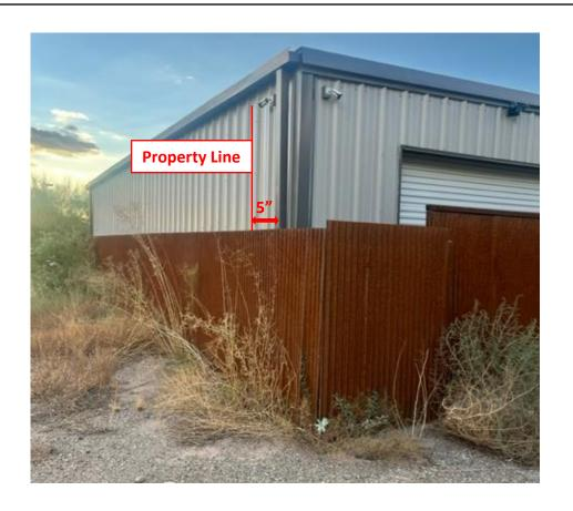
Item 5: UDC Table 6.3-7.A: Dimensional Standards for the NC, RVC & MU Zones. The required perimeter yard setback from the garage to the east property line is the greater of either 10' or 34 of the height of the exterior wall
