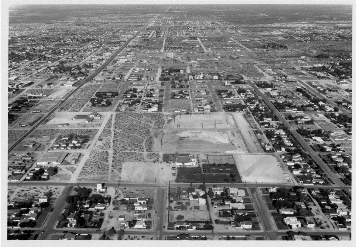
Figure 18: Aerial view of Himmel Park and vicinity, 1940s, looking east. The swimming pool is immediately east of a small, landscaped area (the park at that time). Note the lighted ballfield toward the center of the photo. Farther east the Benedictine Monastery is visible. The water tower on Tucson Boulevard is also visible near the bottom of the photo. (PC 177, A.E. Magee Photo Collection, Box 4, Folder 38, Photo No. 379, Arizona Historical Society Library, Tucson)
