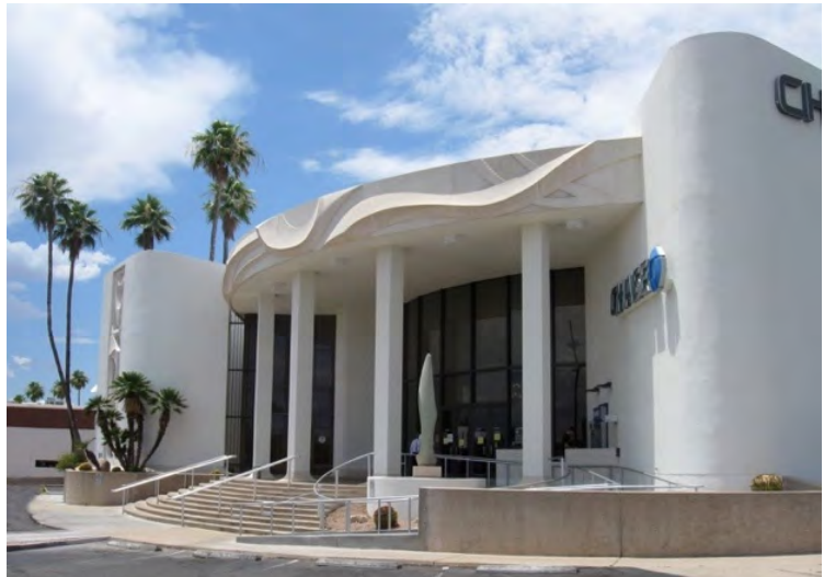
Figure 26: Chase Bank, northwest corner of Broadway Boulevard and Country Club Road.
