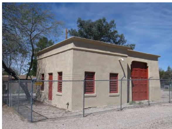
Figure 42: Renovated first floor of water tower on SW corner of 1 st Street and Tucson Boulevard.
