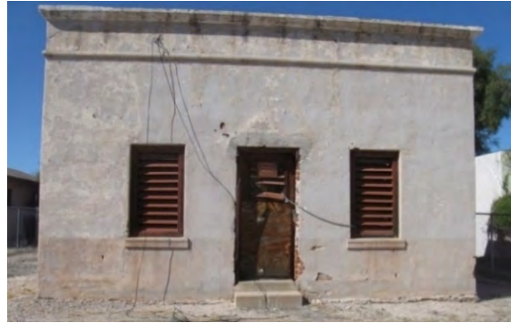
Figure 41: Old water tower at 2218 E. 1 st
