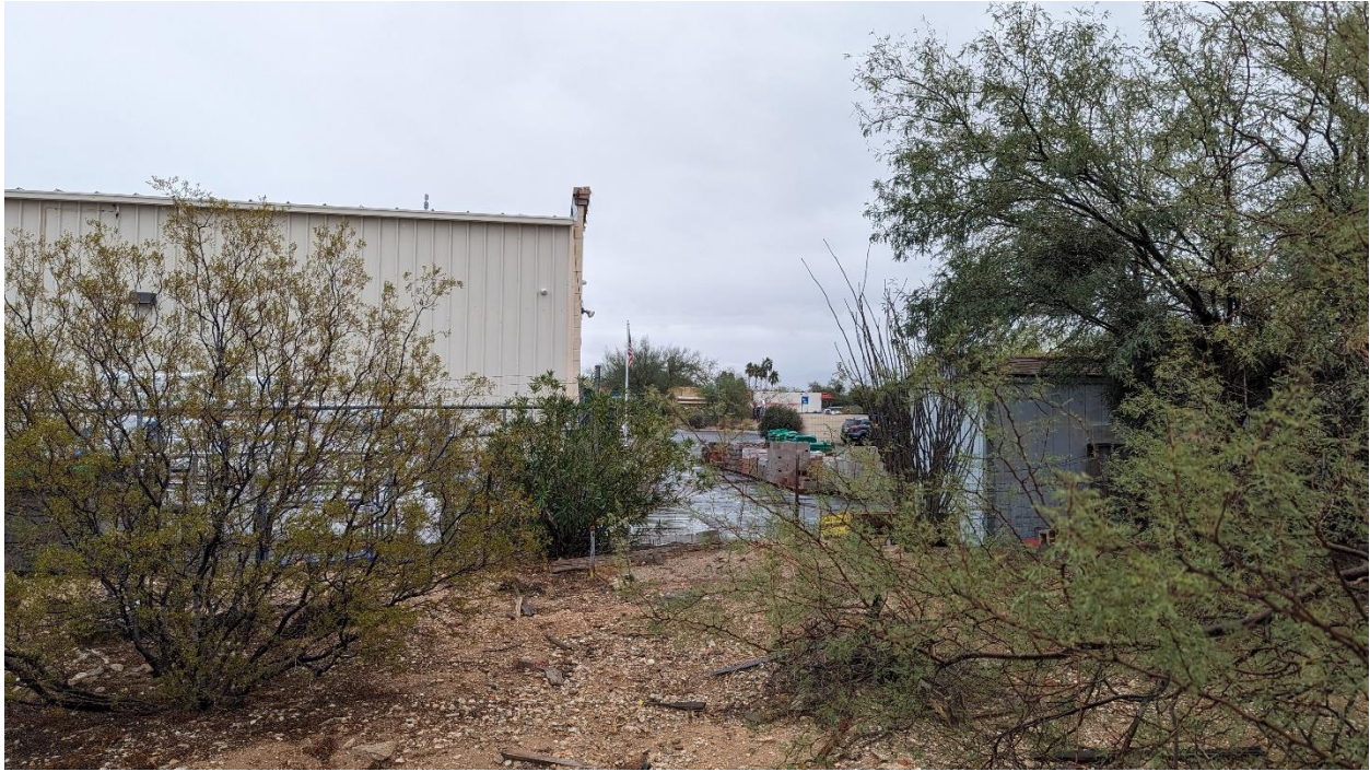
PHOTO #5: View of the backside of the adjacent hardware store from the northeast portion of the site looking east.
