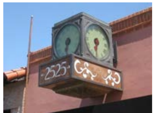
Figure 24: Grunewald and Adams clock above the easternmost store in the Rincon Market complex.
