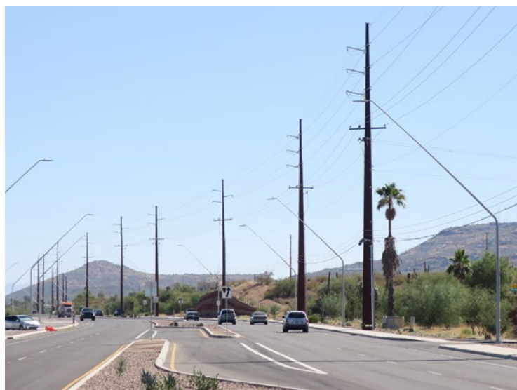
Figure 7.—Silverbell Road and Grant. Weathering steel poles are the dominant skyline feature. Photos by Ellen Barth Alster, used with permission.
