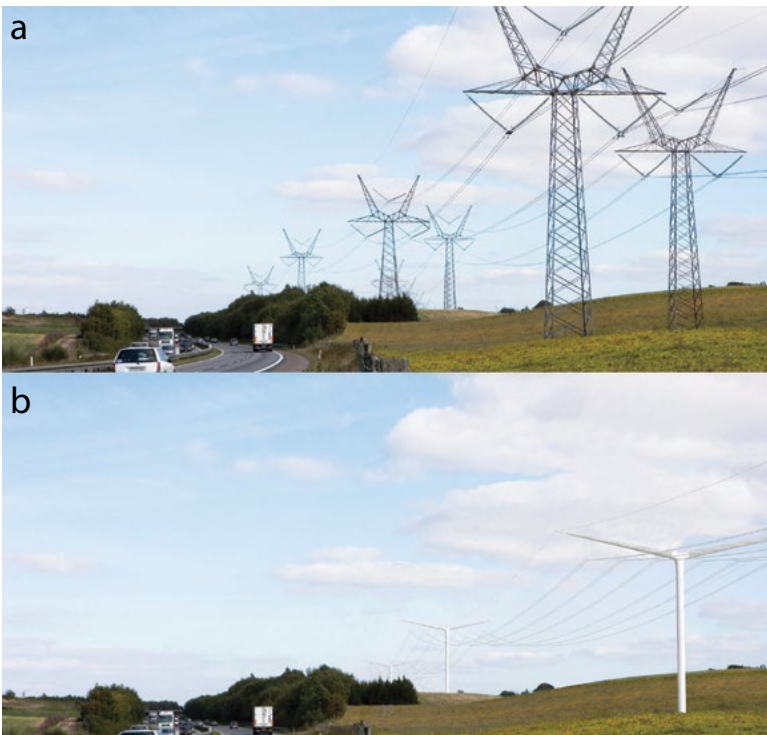
Figure 13.—The composite pylon, currently under development, is half the size of a conventional lattice tower, while carrying the same amount of power. It can be assembled on site and erected in a day. An existing line (a), with two lines each carrying 1x400 kV; the proposed improvement (b) with a single pylon carrying 2x400 kV. (Bystrup 2015). Photos by Bystrup Architects, used with permission.
