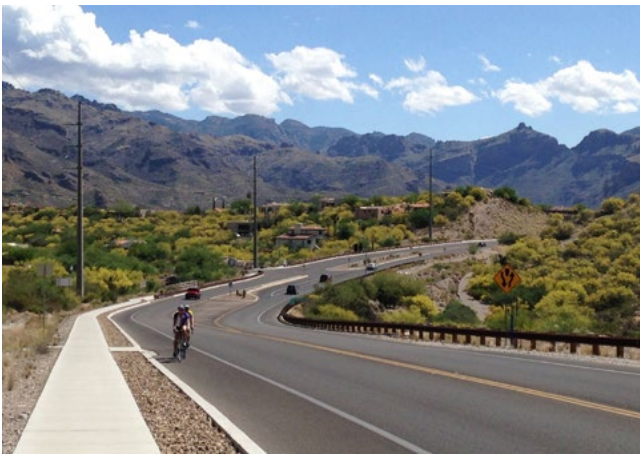
Figure 3—Poles around Tucson used finishes that minimized contrast, receding into the landscape. The practice of painting the poles was discontinued. Photos by Ellen Barth Alster, used with permission.
