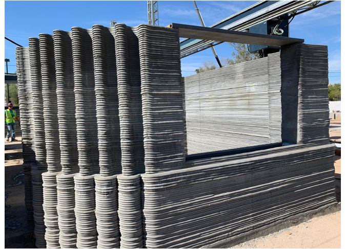
The first home constructed by Habitat for Humanity using 3D printing in Tempe, Arizona
