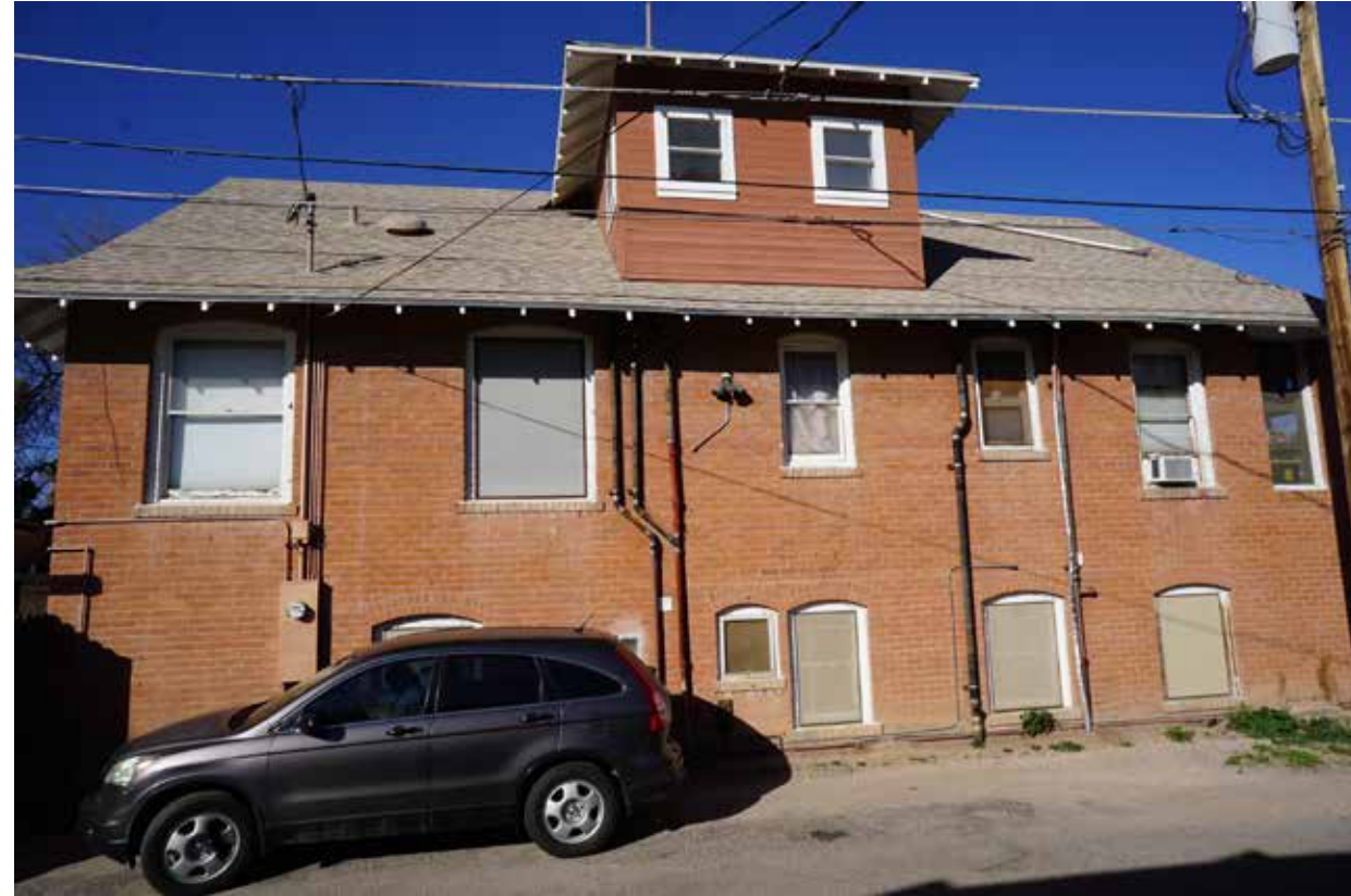
924 N 6TH AVE EAST ELEVATION CONTRIBUTING PROPERTY
