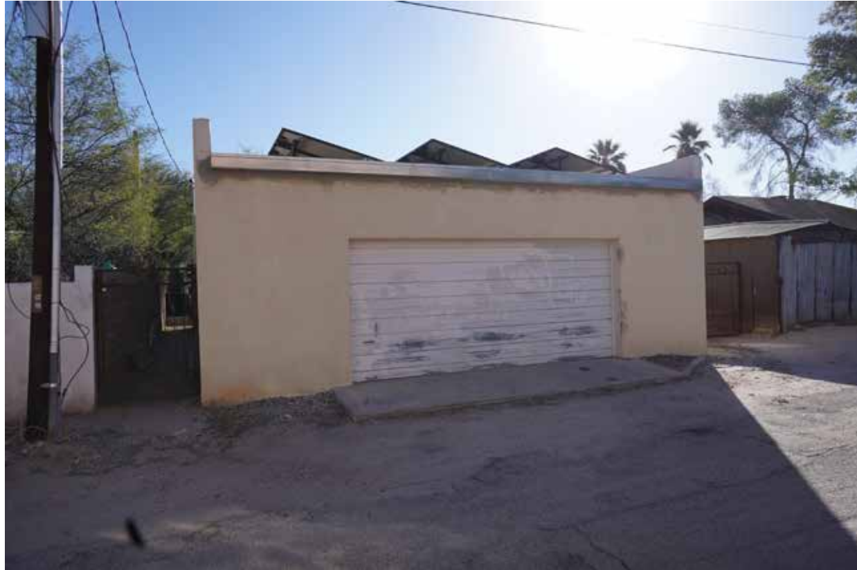
919 N 5TH AVE WEST ELEVATION CONTRIBUTING PROPERTY (GARAGE IS A NON-CONTRIBUTING STRUCTURE)
