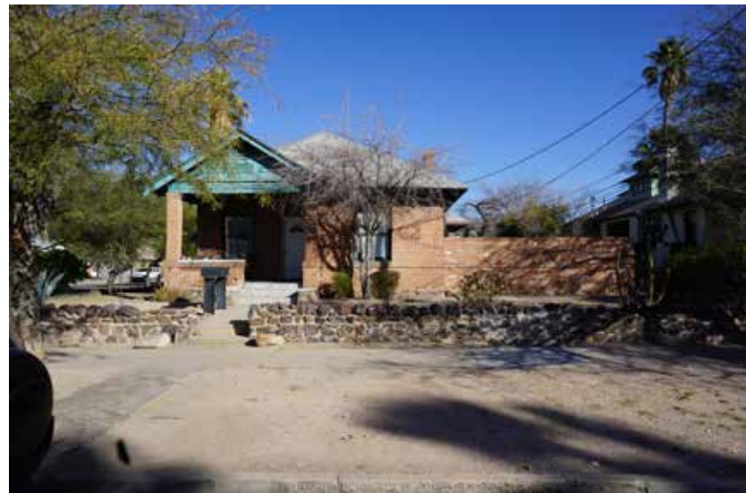
203 E 2ND ST SOUTH ELEVATION CONTRIBUTING PROPERTY
