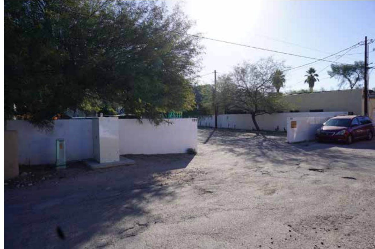
931 N 5TH AVE WEST ELEVATION CONTRIBUTING PROPERTY
