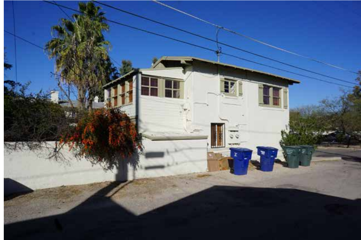
224 E 1ST ST EAST ELEVATION CONTRIBUTING PROPERTY
