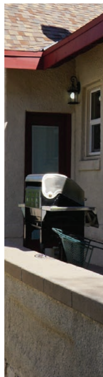
REPLACED DOOR ORIGINAL: BOARDED UP PLYWOOD NEW: WOOD, SINGLE LITE
