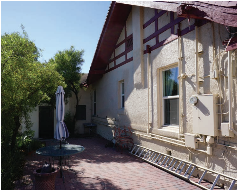
REPLACED ORIGINAL: WOOD FIXED, PICTURE NEW: VINYL FIXED, PICTURE DOOR REPLACED ORIGINAL: HOLLOW CORE WOOD NEW: SOLID CORE WOOD
