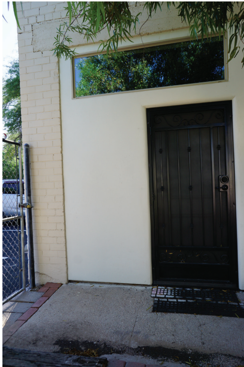
REPLACED ORIGINAL: WOOD FIXED, PICTURE NEW: VINYL FIXED, PICTURE DOOR REPLACED ORIGINAL: HOLLOW CORE WOOD NEW: SOLID CORE WOOD
