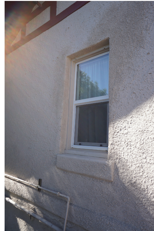
REPLACED ORIGINAL: WOOD SINGLE HUNG, 1/1 NEW: VINYL SINGLE HUNG, 1/1
