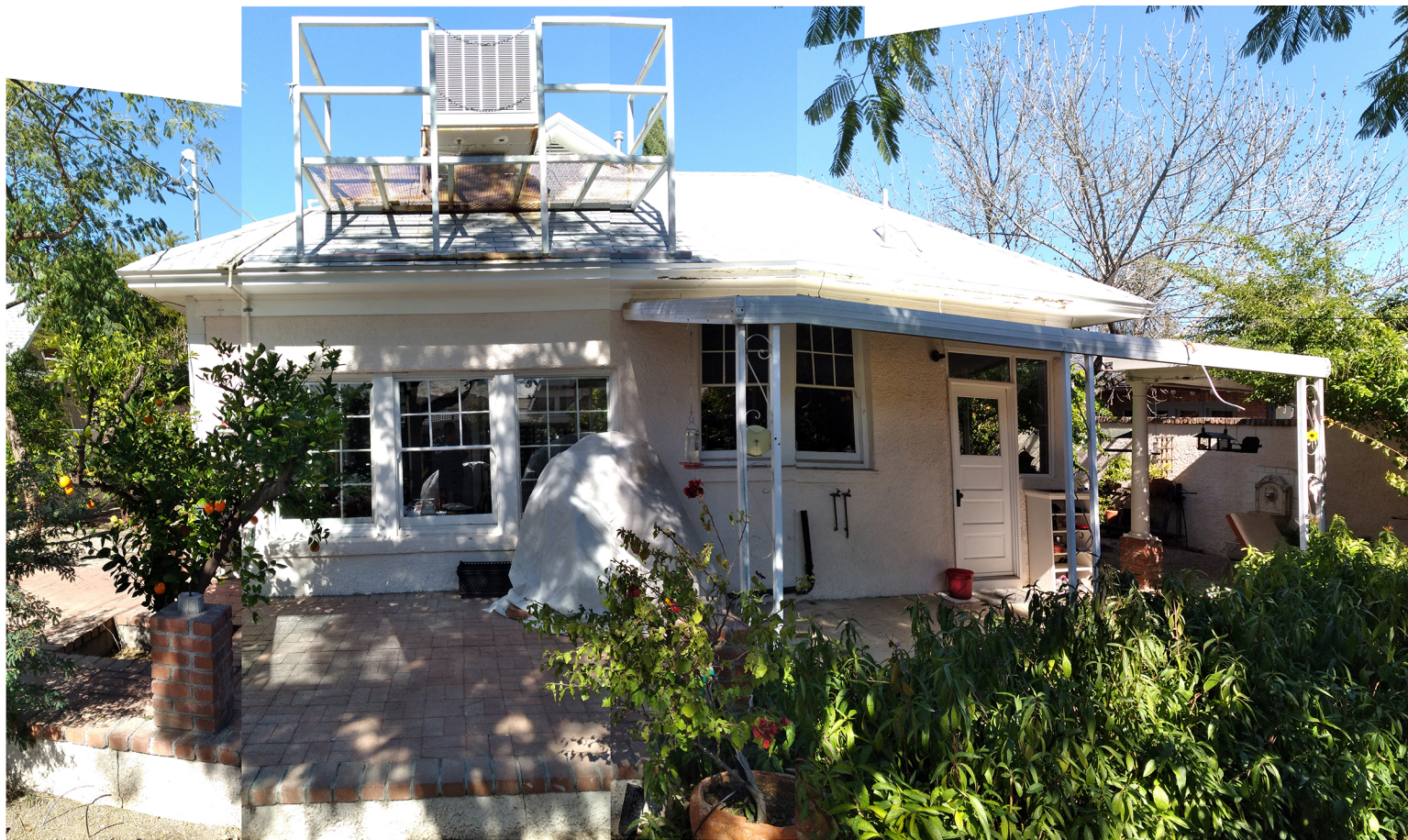
SOUTH ELEVATION - VIEW FROM BACK YARD
