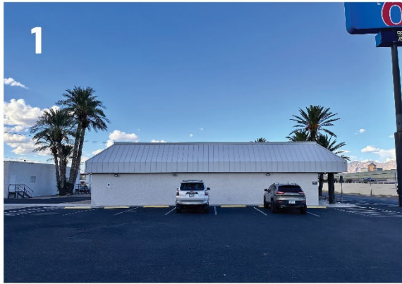
Looking north at south side of Property.
