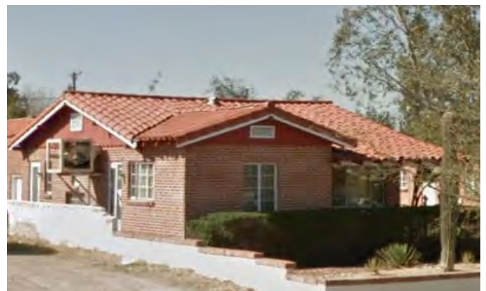
Cross gable roof with clay tile
