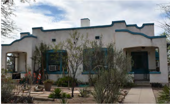
Flat roof with stepped parapet and asphalt
