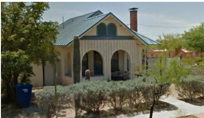
Porch materials and texture are incompatible with the historic district character.
