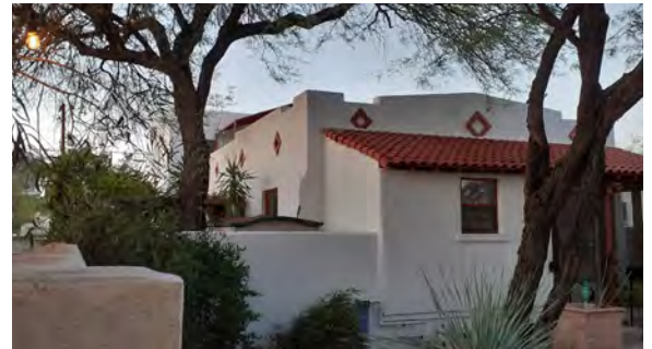
Second-story addition is setback from street, (visible behind left tree)
