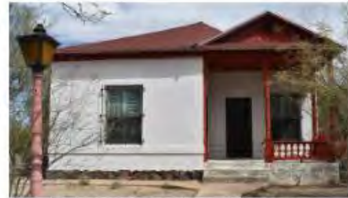
Double-hung sash window with bar guard
