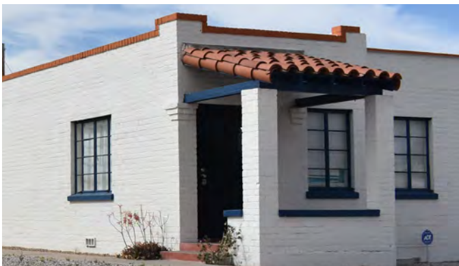
Multi-light casement windows
