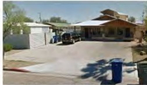
Parking area spans entire front of building
