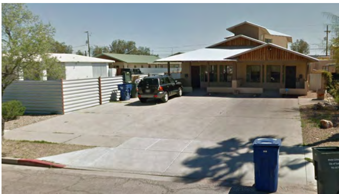
Parking area spans entire front of building
