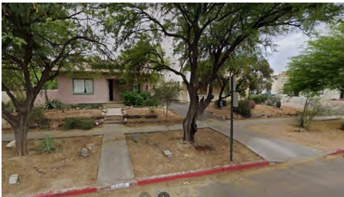
Minimal intrusion of sidewalk with driveway apron
