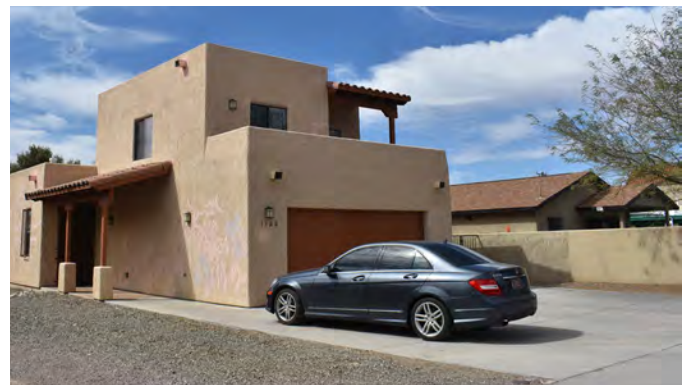
Prominent front facing garage and driveway
