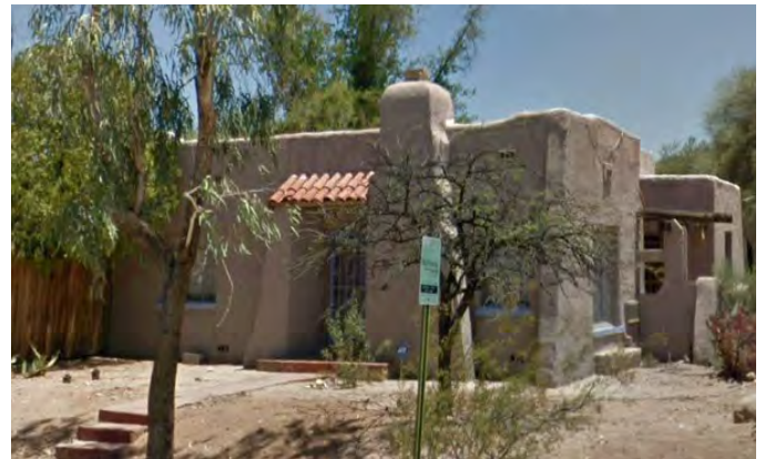
Flat roof with rounded parapet and asphalt
