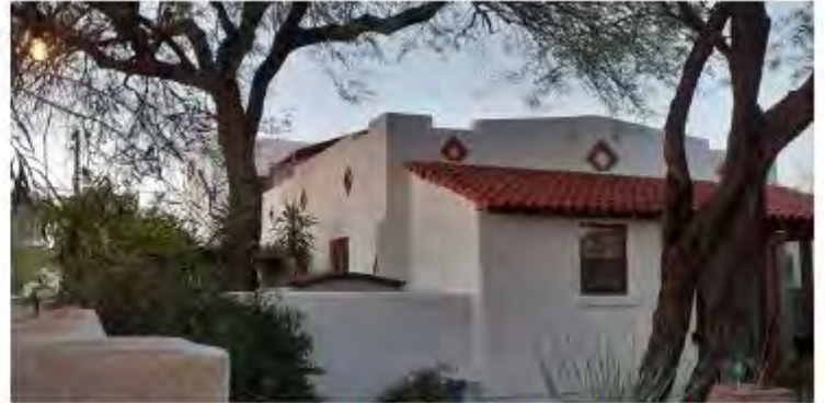
Second-story addition is setback from street, (visible behind left tree)
