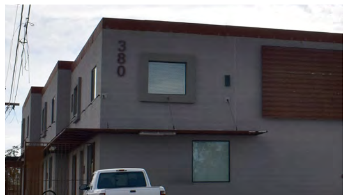
Single-light fixed windows
