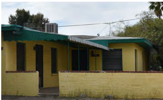
Cross gable roof with prepared roll
