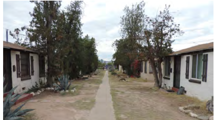
Single-story units set around a courtyard
