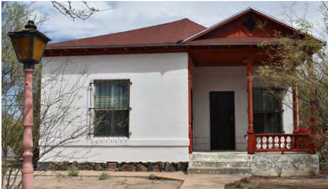
Double-hung sash window with bar guard
