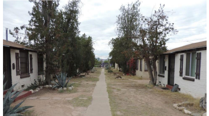
Single-story units set around a courtyard
