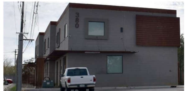
Street-facing details (awnings, wall variations) are articulated to make the building human-scaled
