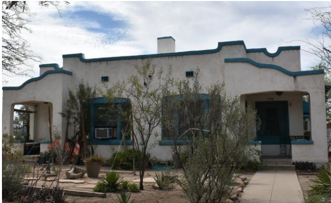
Flat roof with stepped parapet and asphalt
