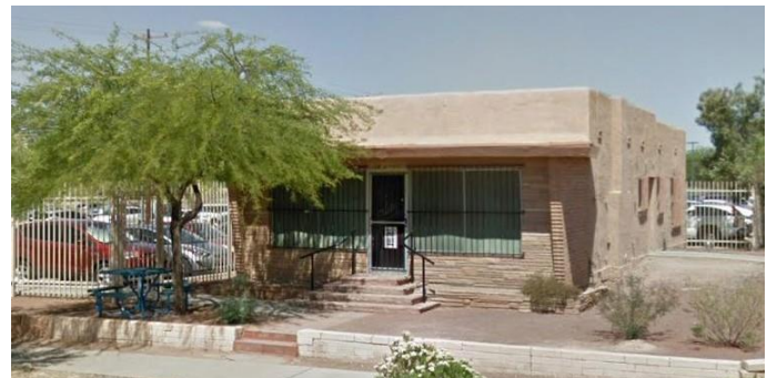
Example of applied façade materials
