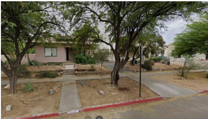
Minimal intrusion of sidewalk with driveway apron
