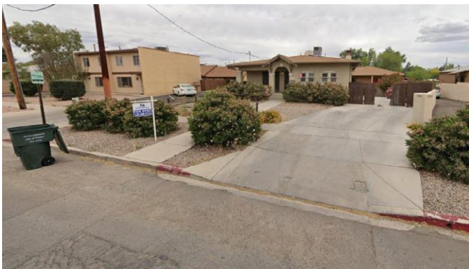
Substantial intrusion on sidewalk with wide driveway apron
