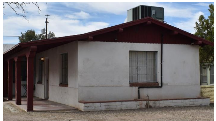
Multi-light steel casement window
