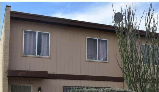
Sliding sash windows, flush with outer wall surface
