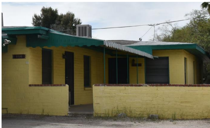
Cross gable roof with prepared roll
