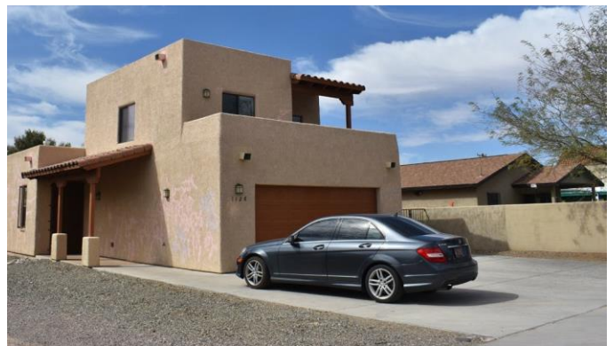
Prominent front facing garage and driveway
