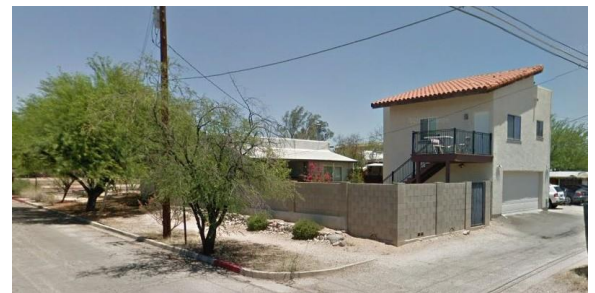
Second-story addition placed at rear of lot; vehicle access via back alley
