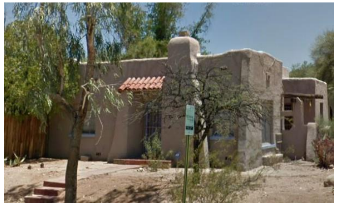
Flat roof with rounded parapet and asphalt
