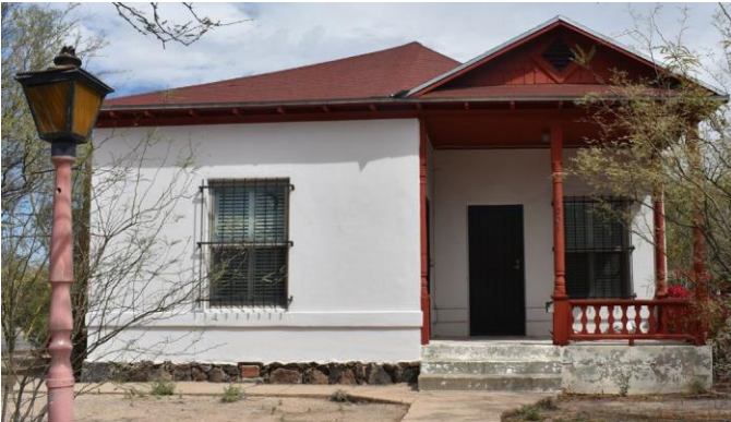
Double-hung sash window with bar guard
