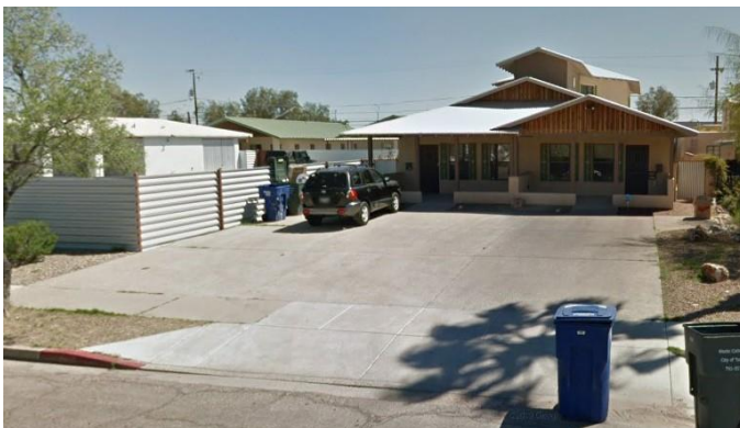
Parking area spans entire front of building
